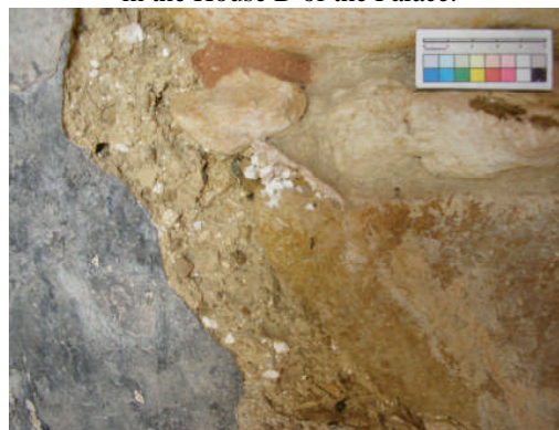
Fig. 7.4. Dividing wall (architectural modification) at the Temple of the Foliated Cross. Mud plaster with unmixed lime lumps. A limewash painted on black can be seen at the left.
