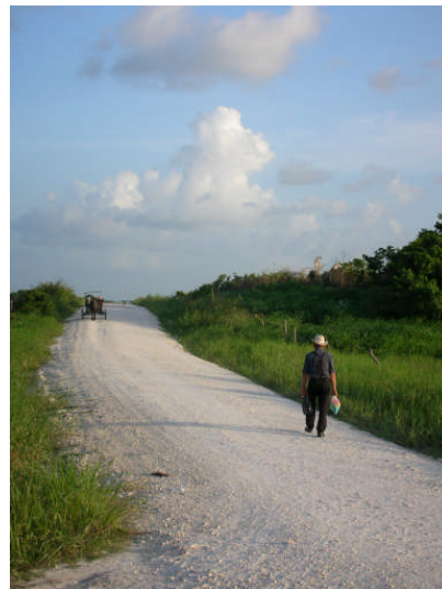
Fig. 7.25. Construction of sascab roads in Belize, close to the site of Lamanai.
