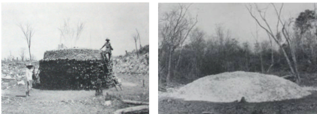
Fig. 3.8. Left: Calera construction in the early 20 th at Chichén Itzá. Right: After the burn the lime is left to slake in the open air. Pictures: Morris and colleagues (1931).
