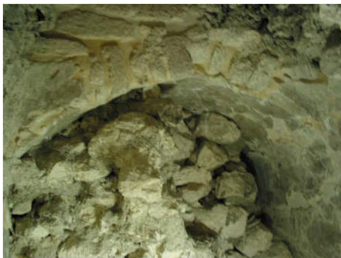
Fig. 2.16. Barrel vault of Substructure IIc, showing later fill. Image: Rodríguez Campero2008.
