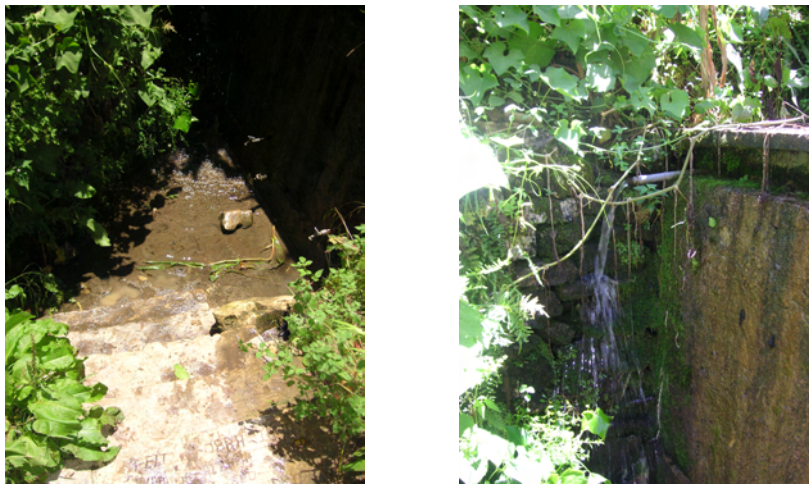
Plate 9 Steps down to taps (left) and overflow pipe (right)
