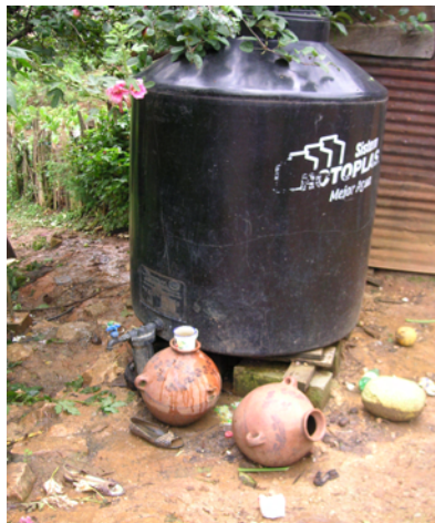
Plate 4 Example of a 1,700-litre tinaco, commonly used for water storage across Mexico
