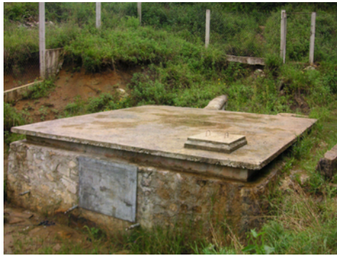
Plate 7 Main spring box (left) and adjacent overflow area (right)
