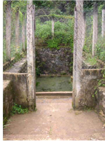
Plate 7 Main spring box (left) and adjacent overflow area (right)
