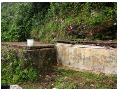
Plate 8 Spring boxes (left) and interior of right-hand spring box (right)
