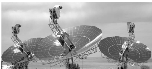
Figure 2. Dish-Stirling system. SES (Stirling Energy Systems) prototype .
