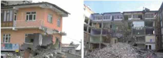
Figure 15. Damage due to the impact of the collapsed building on the neighbouring building in Erciř and Van
