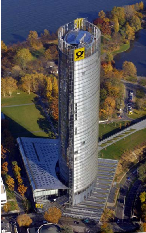
Figure 1. Post Tower. Photograph courtesy of Deutsche Post AG (2003).
