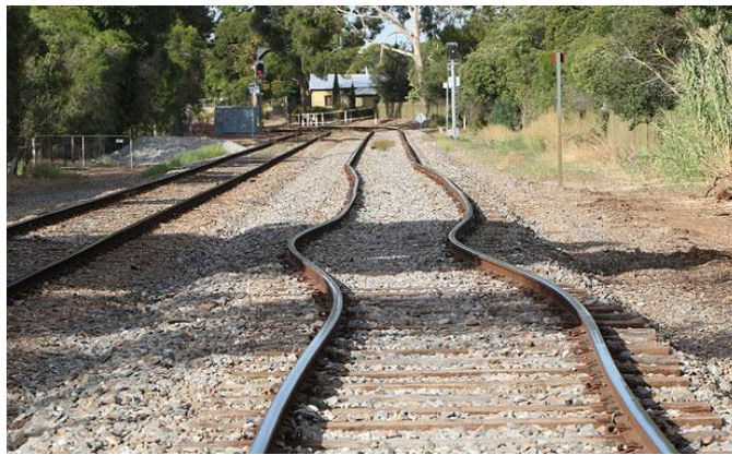
Figure 1.1 Thermal Buckling in a Continuous Welded Rail (Robertson 2012)
