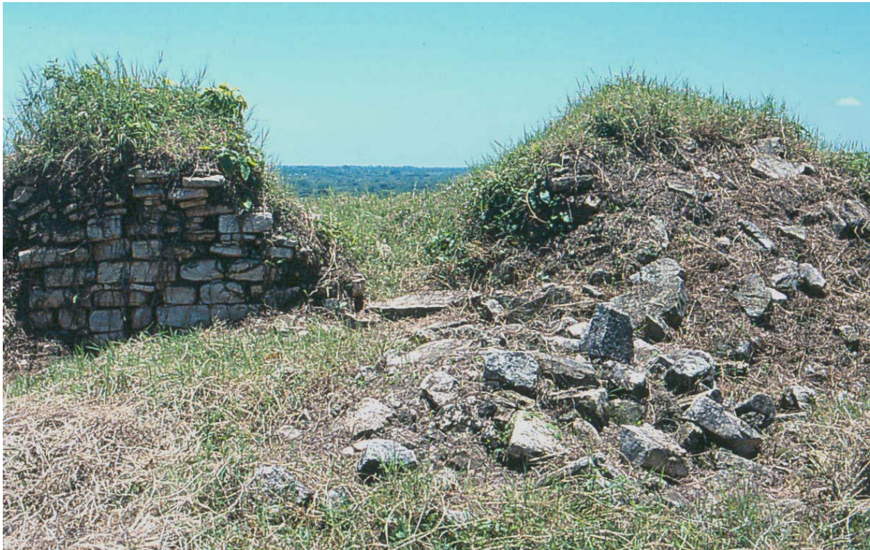
Figure 2.9: View of Structure 3 remaining walls
