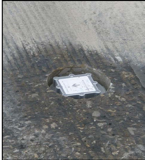
B – Detail of the sensor ready to be covered with epoxy.
