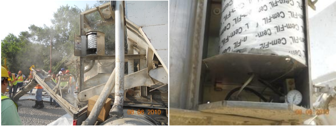
Figure 4.4. Fiber feeder system adapted to the mobile trucks.
