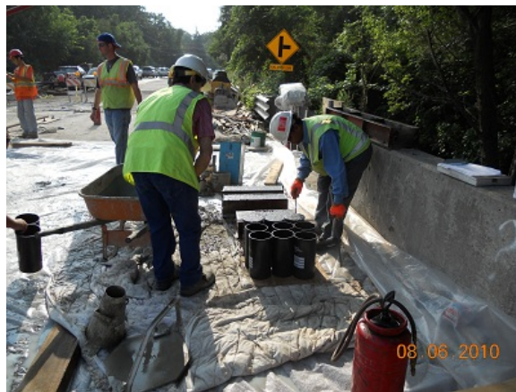
Figure 4.8. Quality-control practices and preparation of the LMC overlay test specimens.
