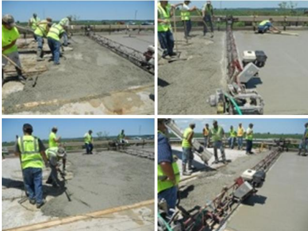
Figure 4.17. Placement of the fibrous FAC overlay.
