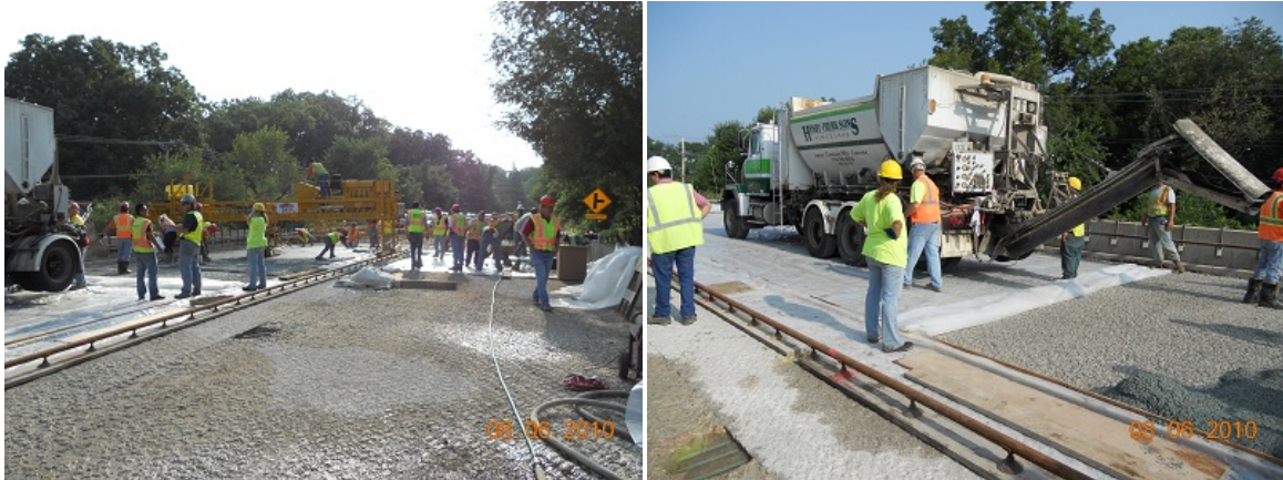
Figure 4.2. Construction site with the contractor and IDOT crews (LMC overlay).
