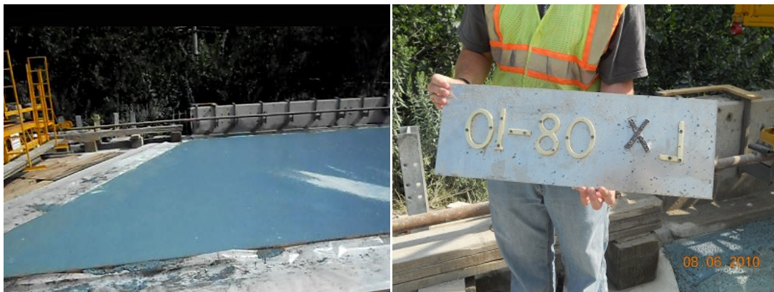
Figure 4.11. Finished surface of the fibrous LMC overlay ready for the stamp.
