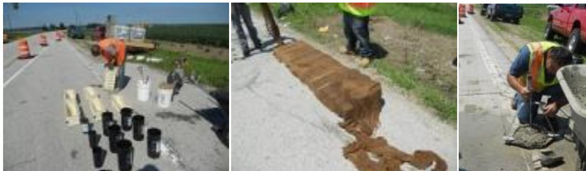
Figure 4.19. Quality control and preparation of the fibrous FAC test specimens.
