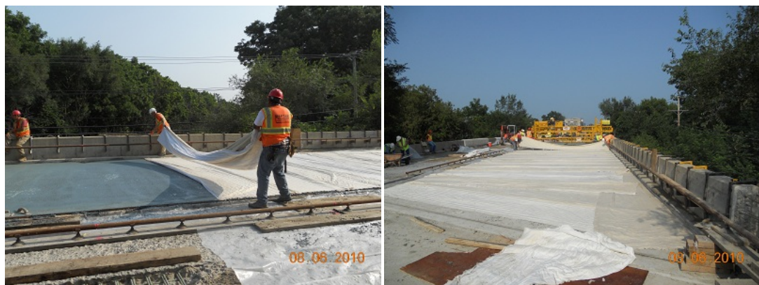
Figure 4.12. Laying down the cotton mats for curing of the LMC overlay.
