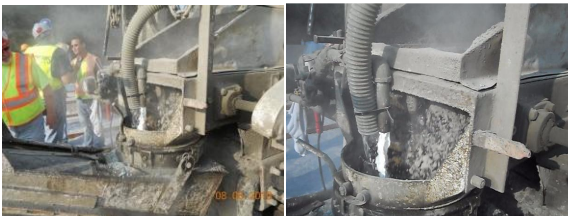
Figure 4.6. Blowing the chopped fibers into the LMC using a pipe under pressurized air.
