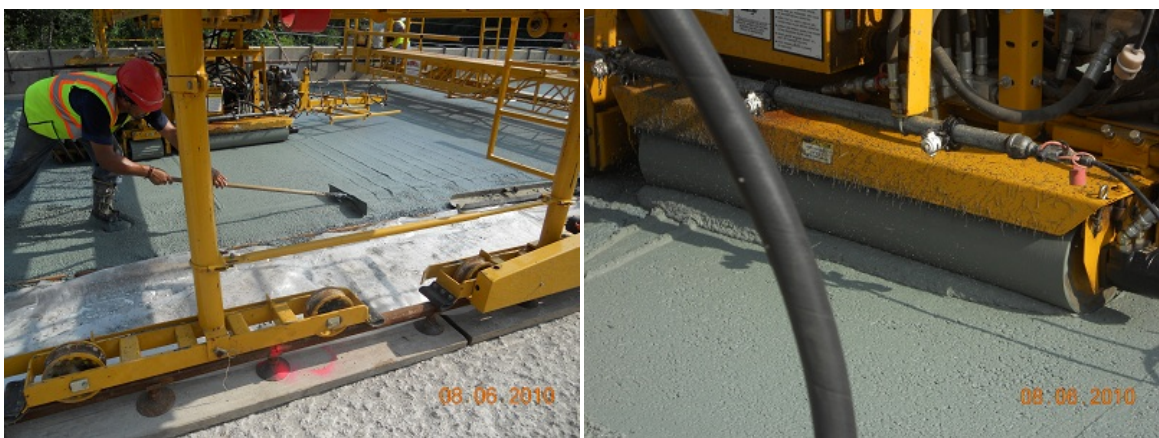
Figure 4.9. Finishing practices of the fibrous LMC overlay.
