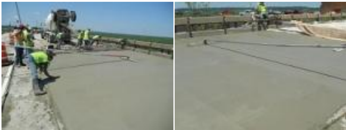
Figure 4.18. Finishing of the fibrous FAC overlay.
