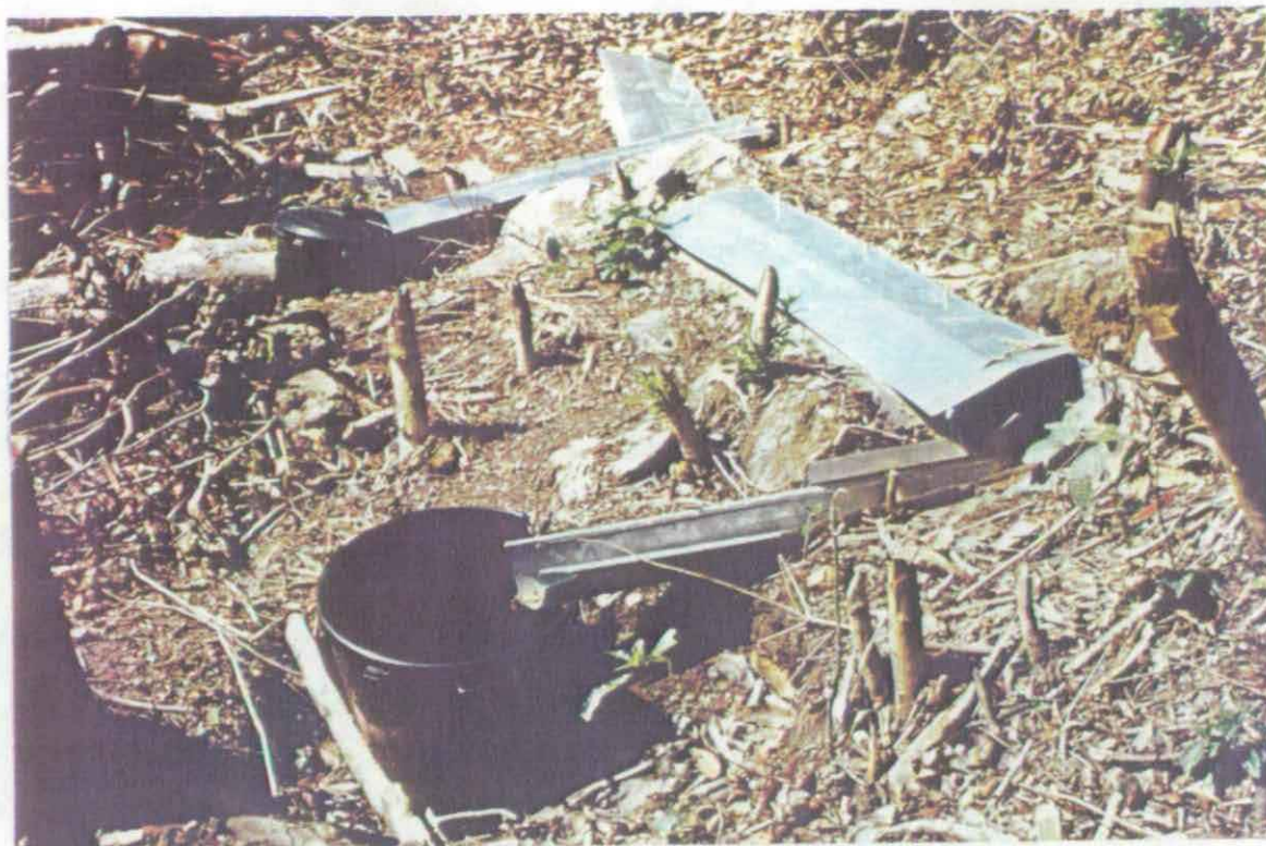
Fig.7. Trough and gutter complete with collecting bucket. The buckets are covered, and some are fitted with overflows.
