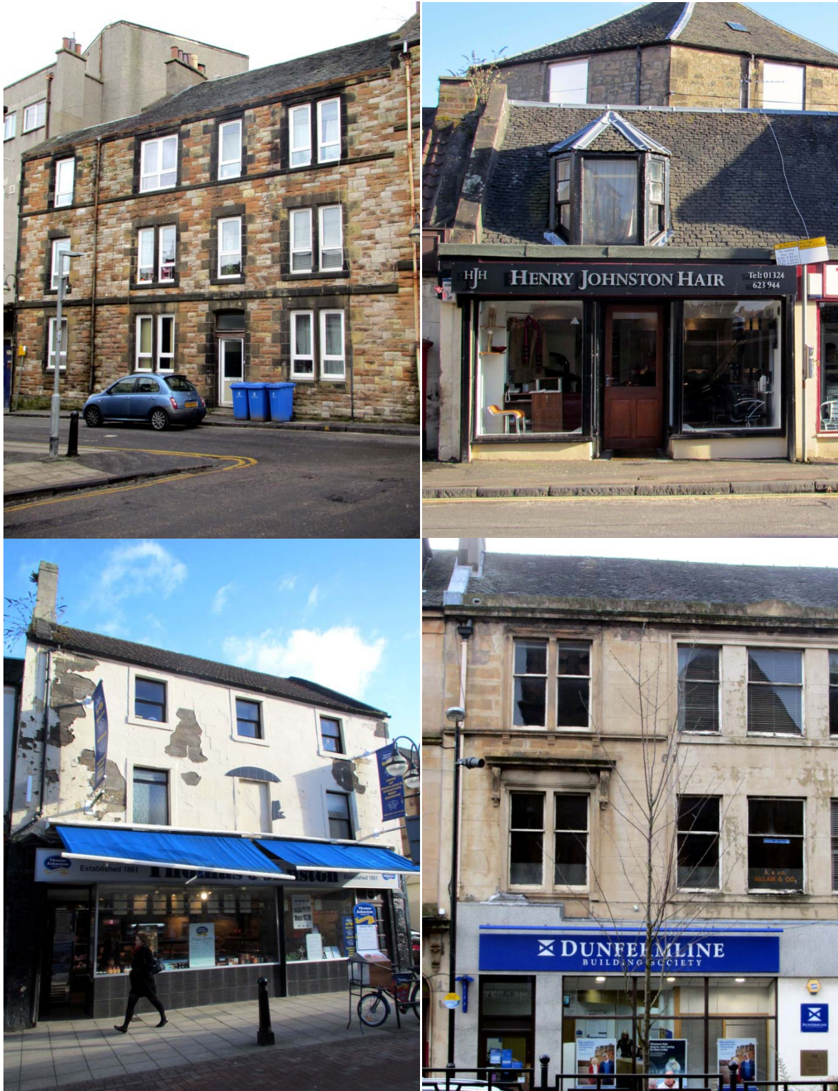
Figure 8 Examples of ‘good’ and ‘poor’ visibility in surveyed Falkirk buildings
