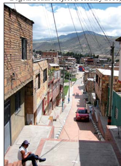
Caracas Sector, after the completion of work to upgrade the infrastructure financed by the Bogotá South Project (August 2004).
