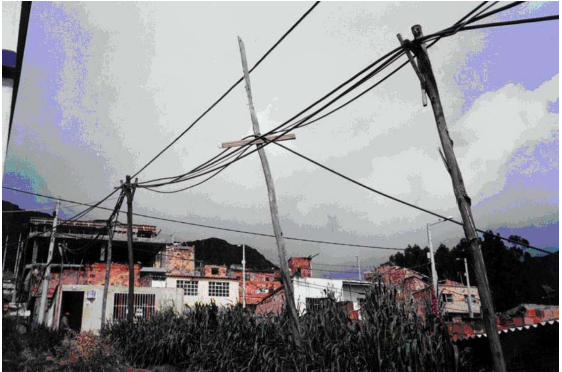
Photograph 2. ' Aeroducto ' (hose connection of water supply in the air) built by communal work in JJR (November 1999).
