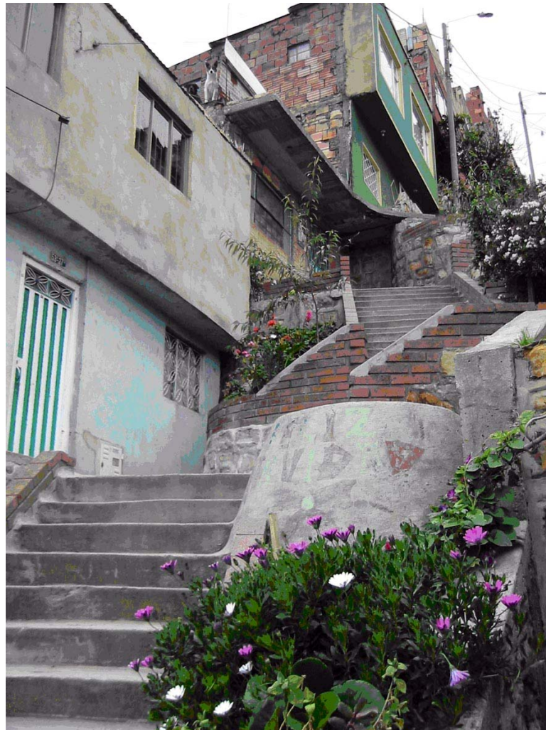
Photograph 6. Steps built by 'OSP' in La Paz (August 2004).
