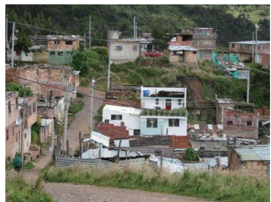
An example of consolidated houses in the first sector (August 2004).
