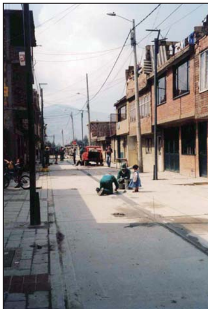
Finishing the pavement (June 2000).
