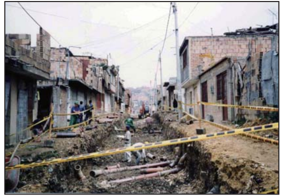
Installation of sewerage system financed by the de-marginalisation programme (February 2000).
