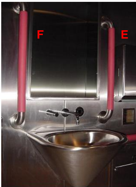
Grab rails E and F. (Bichard 2004) VivaCity 2020
