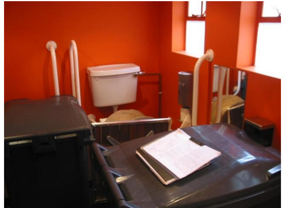
A clip board is also recommended for carrying out toilet audits as some facilities may not have flat surfaces to write on. (Goodwin 2005) VivaCity 2020
