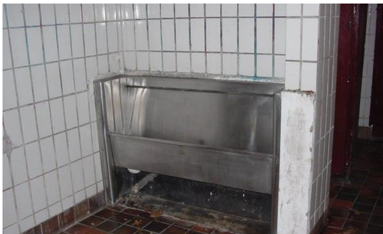
Urinals can be difficult for young boys to use. (Photo courtesy of David Knowles, Bradco/W&G Sissons Ltd 2003) VivaCity 2020
