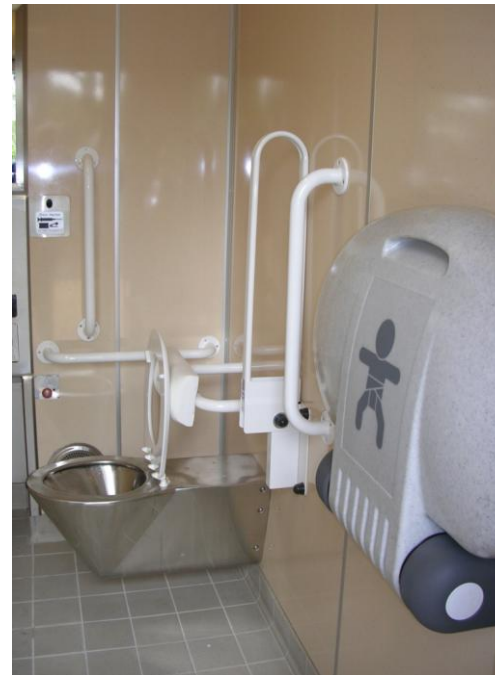
Combined accessible/baby changing facility. (Richard 2003) VivaCity 2020
