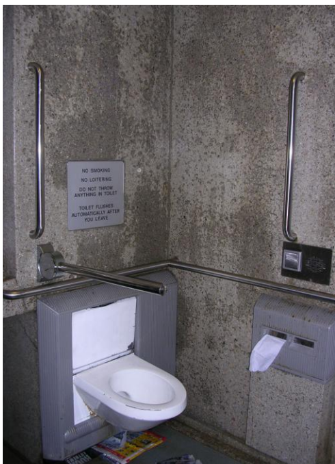
Internal fixtures and fittings of the APC do not match recommended guidelines. (Richard 2005) VivaCity 2020
