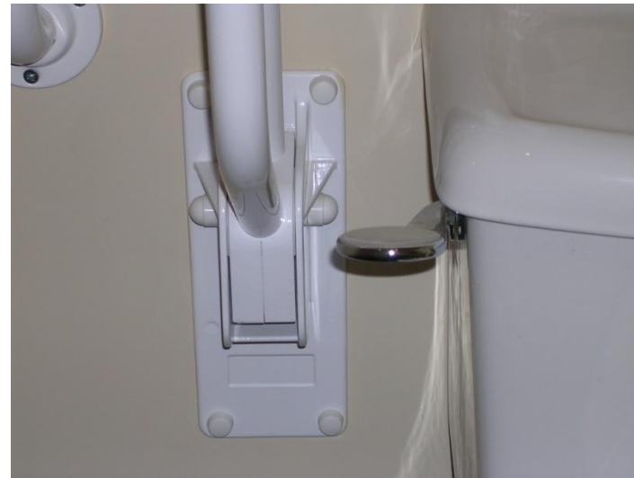
The paddle flush is on the transfer side. (Bichard 2005) VivaCity 2020
