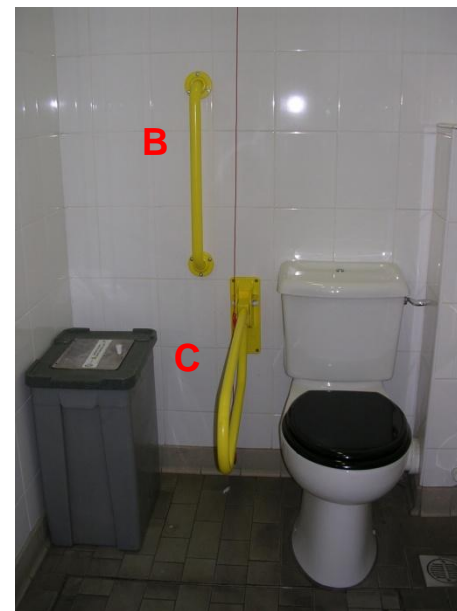
Grab rail B. Note bin incorrectly placed in transfer space. (Bichard 2005) VivaCity 2020
