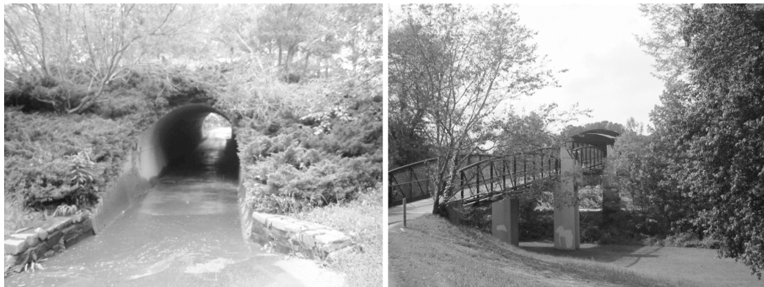
Figure 3. View of a Typical Cart Path Tunnel and Bridge Crossing
