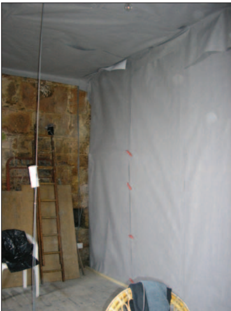
Figure 9 Partitioning of the tower: (above left & middle) wall adjacent to north-west box room and stairway; (right) ceiling south-east corner.
