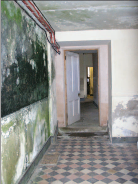
Figure 1 North-east wall of basement
