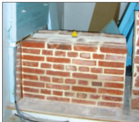
Figure 2 Warm face of brick wall
