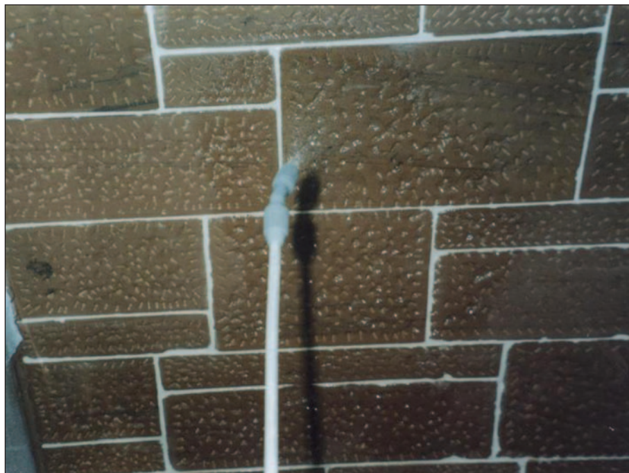
Figure 28 Spraying of stone wall
