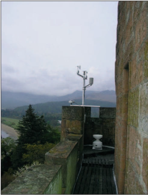
Figure 3 Weather station south-west corner of parapet of Tower
