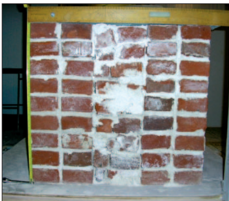
Figure 1 Side view of brick wall
