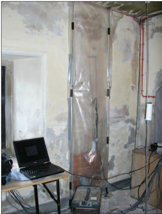
Figure 10 Enclosure and de-humidifier.
