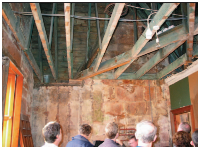
Fig. 2 Tower interior – west wall and roof
