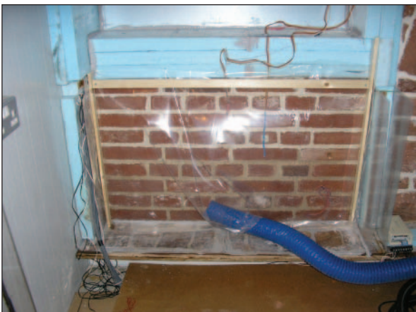
Figure 21 Polythene enclosure covering warm side of brick wall
