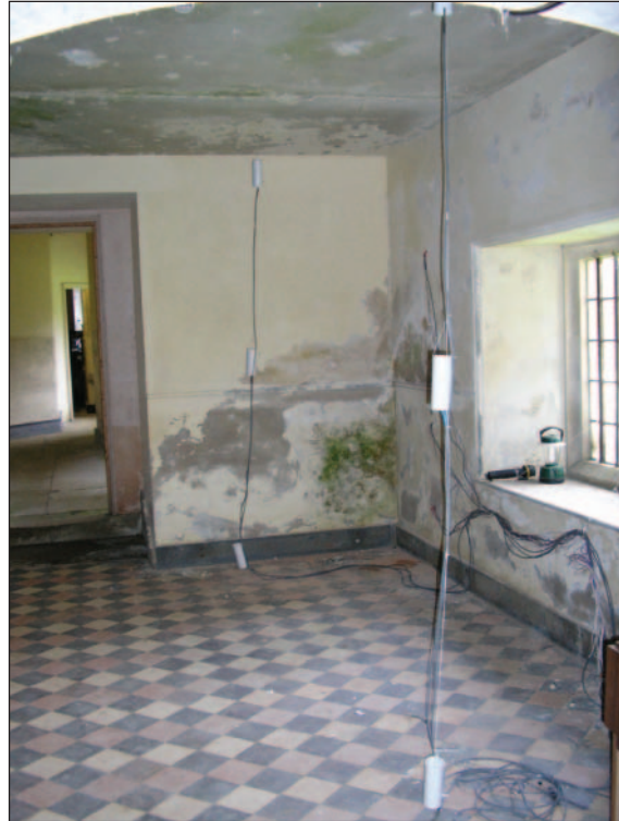
Figure 2 South-west wall of basement
