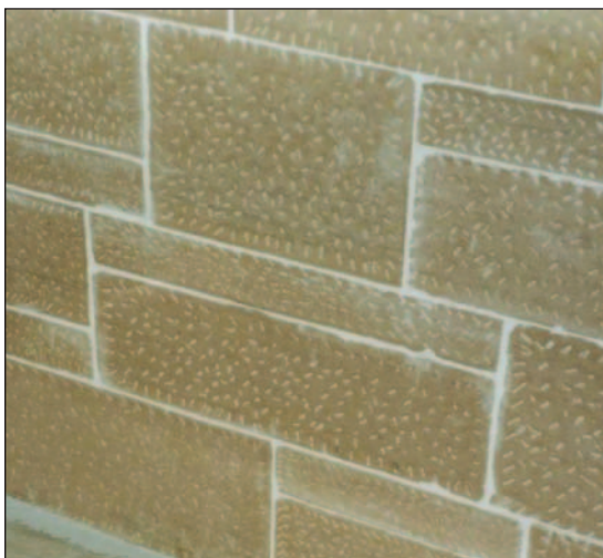
Figure 3 Ashlar finish on cold face of stone wall
