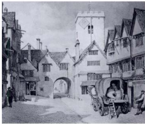
THE NORTH GATE AND ST. MICHAEL'S CHURCH Source: Tyack 1998 (The Church and tower still exist)
