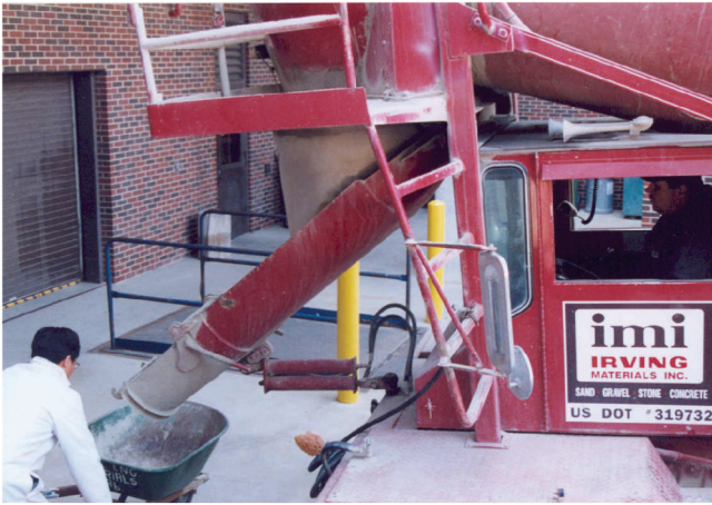
Figure 4.26 Concrete truck parked outside the Civil Engineering Building during concrete delivery.
