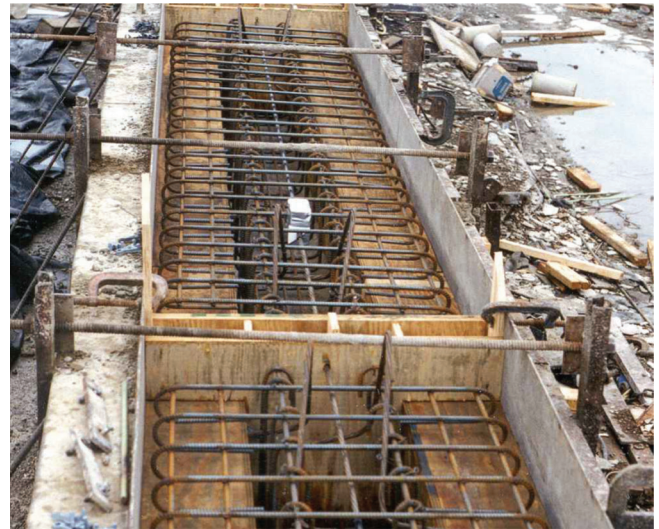
Figure 3.39 Formwork for multiple-strand development length specimens.
