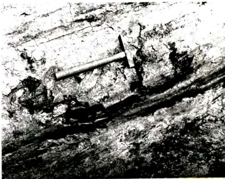
Fig. 98. Gouges developed along the footwall contact.
