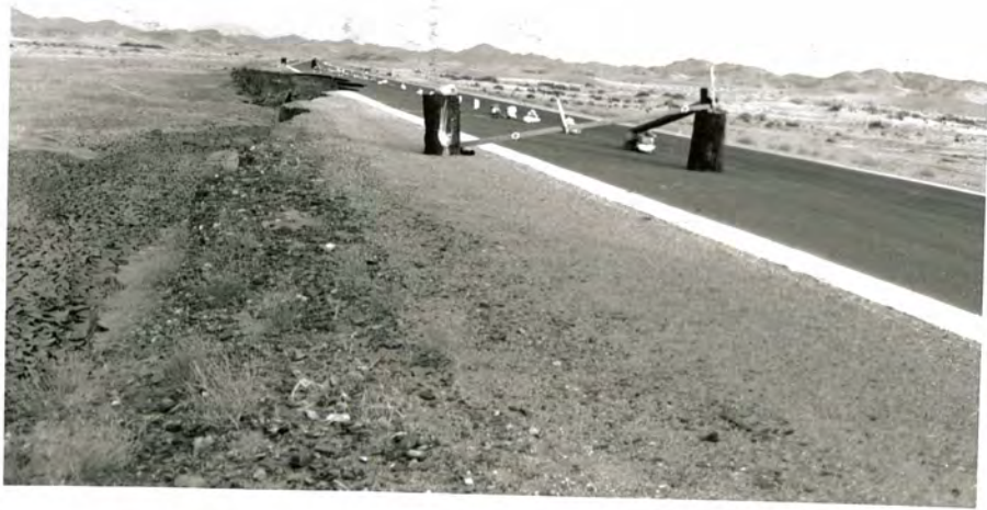
(c) The Mecca Deviation ( Jeddah - Taif road )
