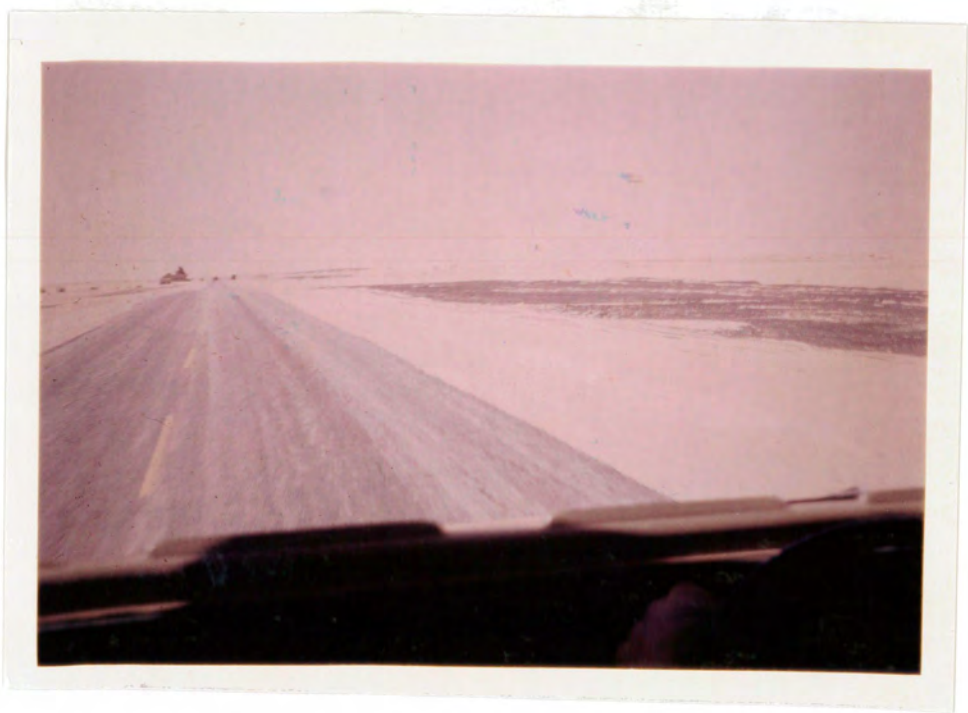
Fig. 4.12 Oil spraying is used to protect the roads from drifting sand. ( The two photographs are for the Riyadh - Dammam road. ).
