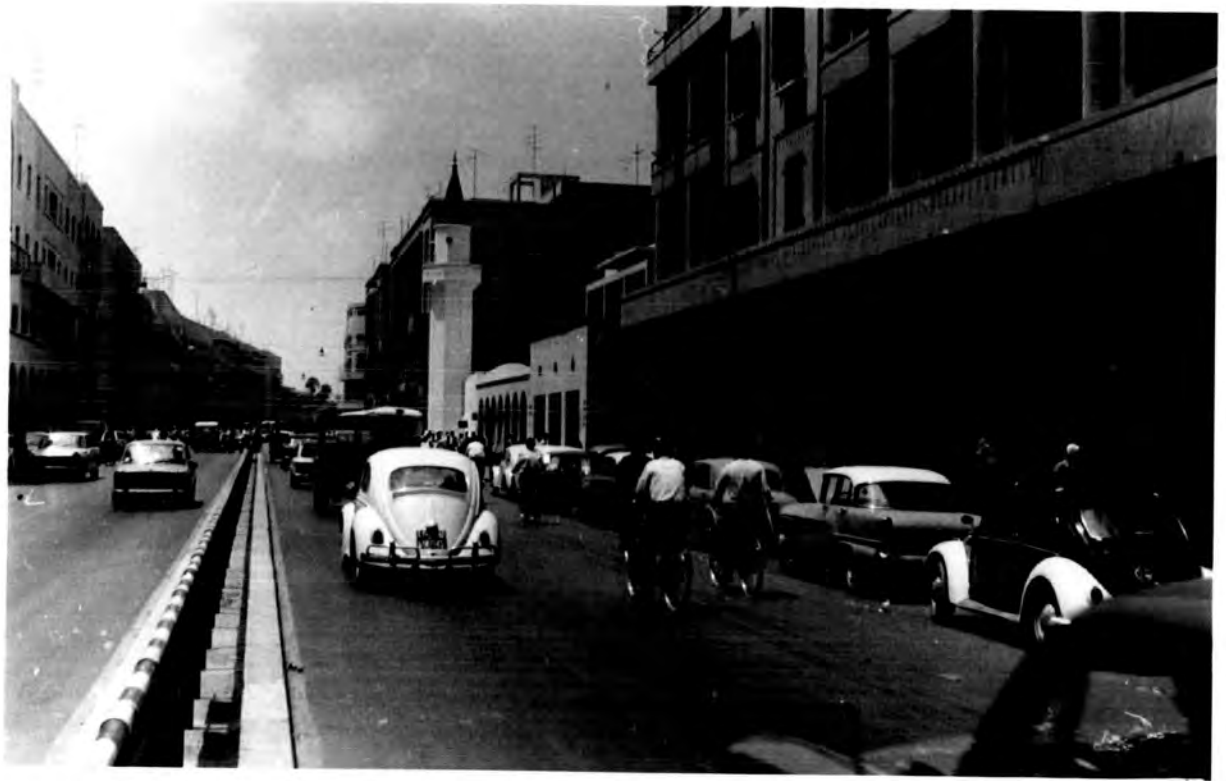
Plate 4.5 Modern shopping centre in Omar el Mukhtar street
