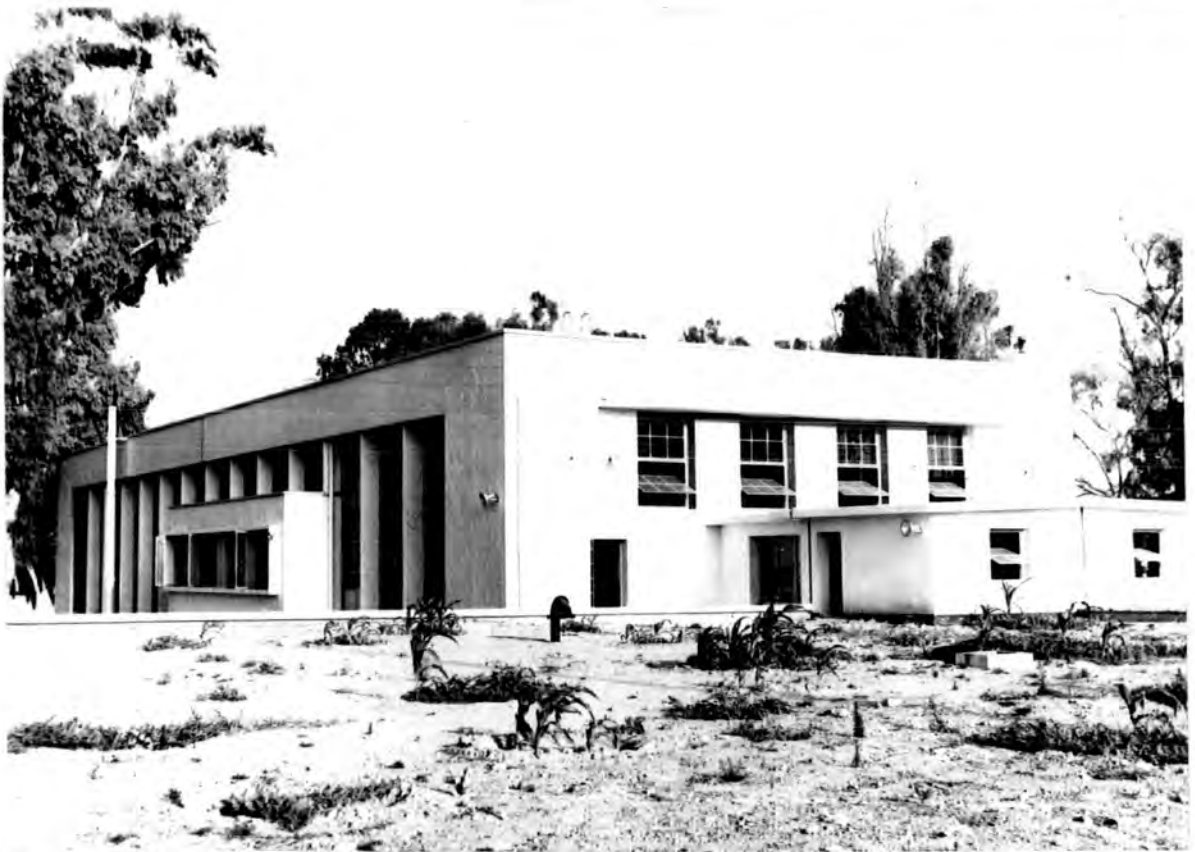
Plate 1.2(A) Bu Mulyana Water Pumping Station
