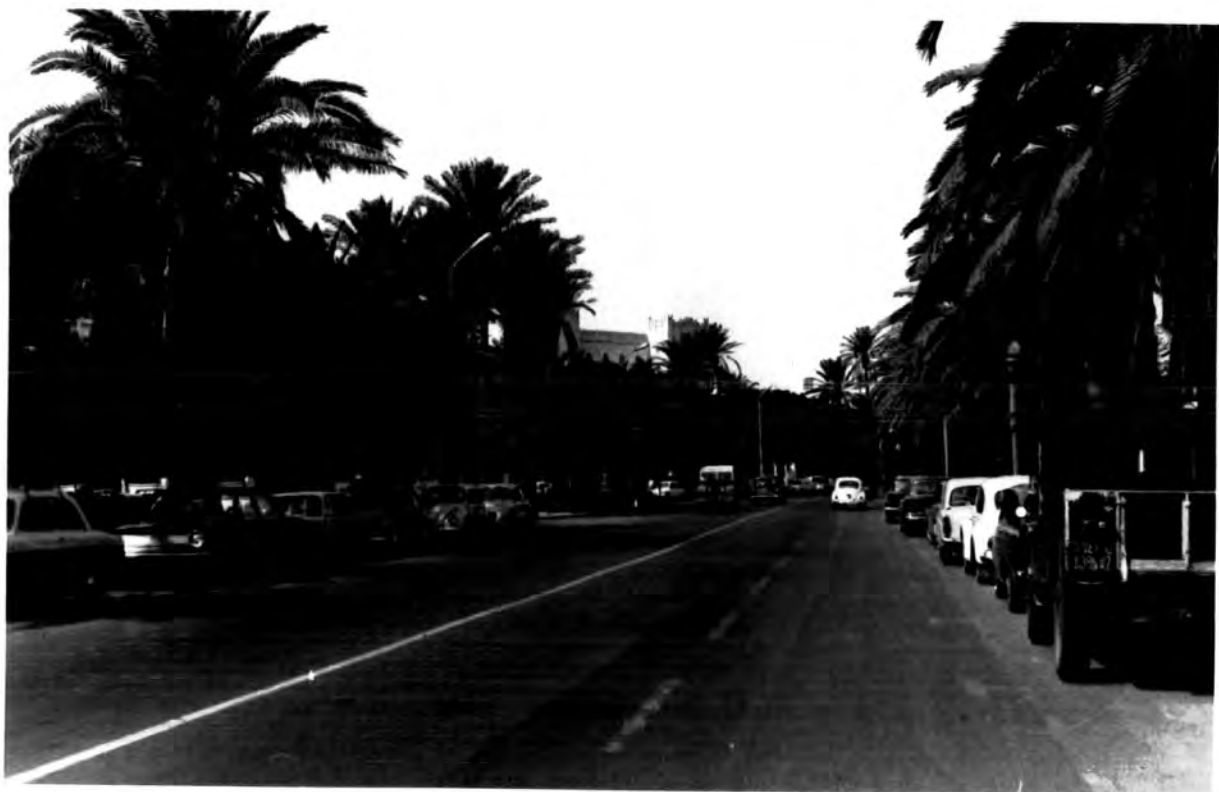
Plate 5.6(A) Adrian Pelt street : northern section. Note the street parking.
