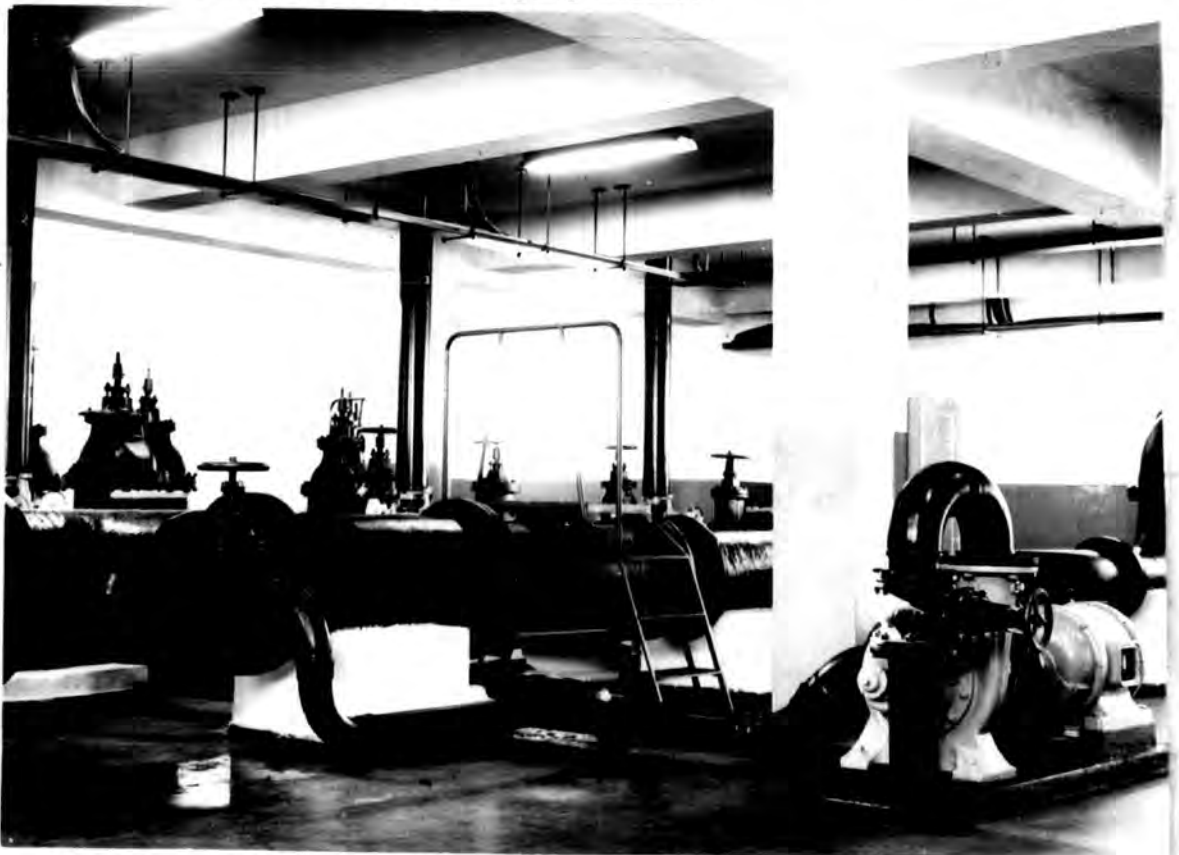
Plate 1.2(B) Bu Mulyana - view of pumping machinery
