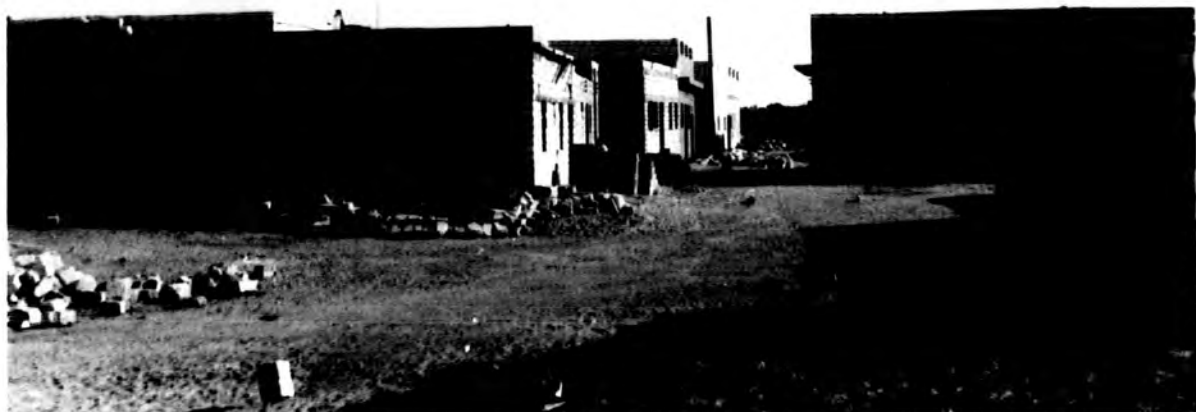
Plate 6.2 Construction of traditional houses in Gurgi
