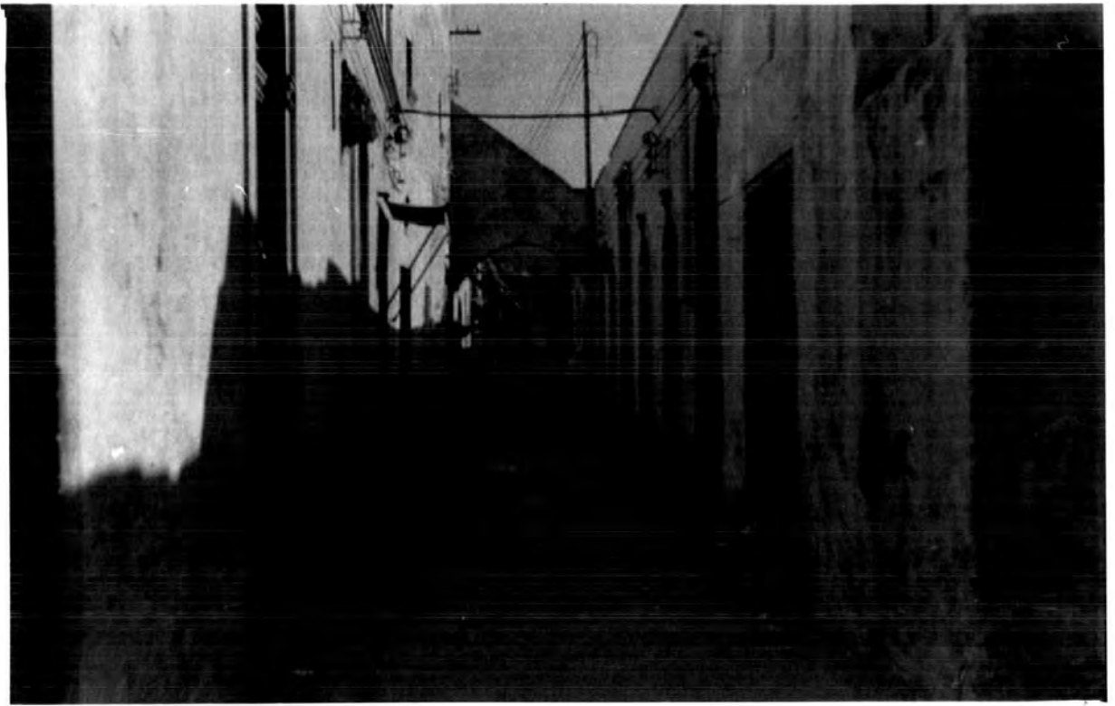
Plate 6.7(A) Semi-derelict houses in Zenghet el Fenedga - Old Town
