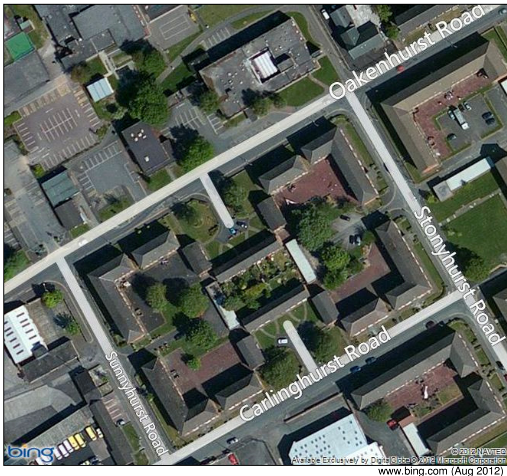
Figure 7.36 Oakenhurst Road, Blackburn – aerial view
