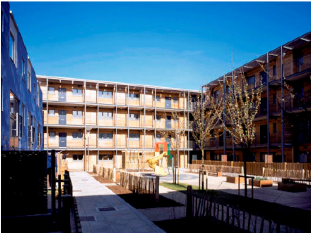
Figure 7.2 Cooper's Road, Southwark, London – inner courtyard
