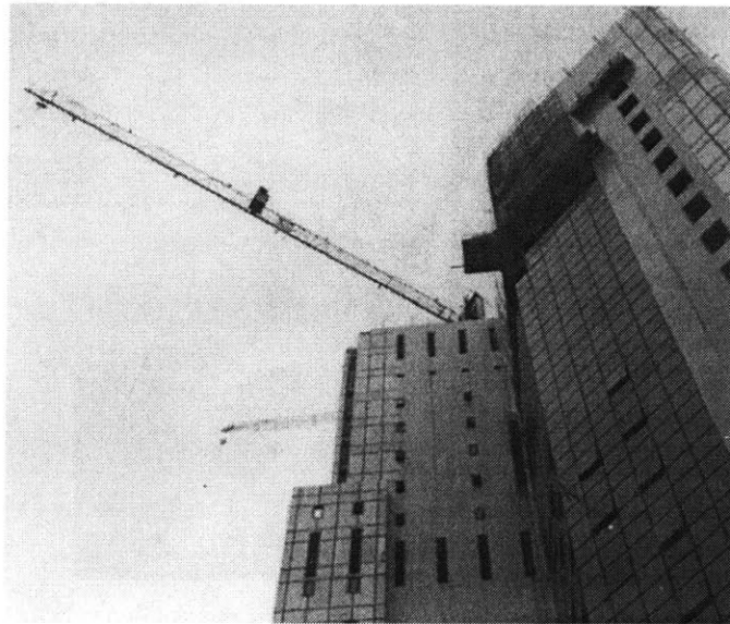
Figure 22 Climbing crane located within the building
