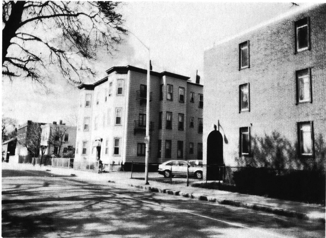
Fig. 4.28 Existing Brick Apartment Building as seen from Putnam Street
