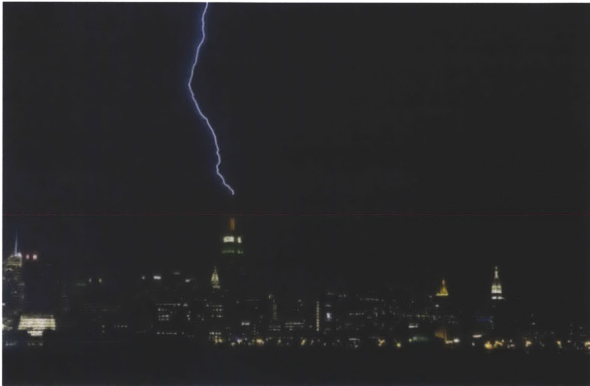
FIGURE 7-9: EMPIRE STATE BUILDING STRUCK BY LIGHTNING
