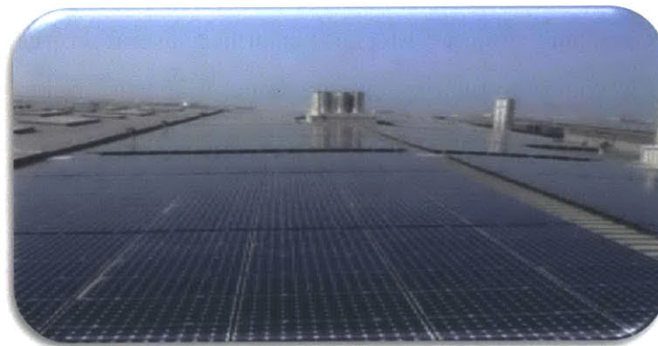
Picture 2: Top Roof PV Installation at KAUST 6
