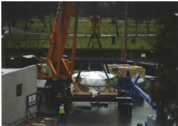
Figure 1.5 – 220 ton isochronous cyclotron being delivered to a new proton therapy facility in Seattle WA
