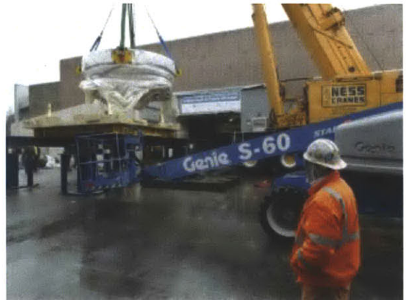
Figure 1.5 – 220 ton isochronous cyclotron being delivered to a new proton therapy facility in Seattle WA
