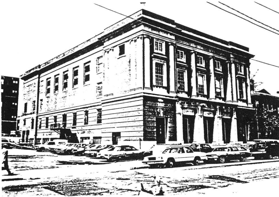
Figure 4-1: Exterior front and side elevation photograph.
