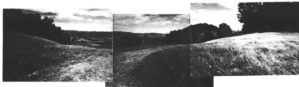
the building site
