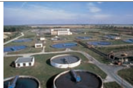
Wastewater treatment in Hungary
