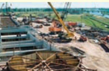
Construction of HSL-Zuid
