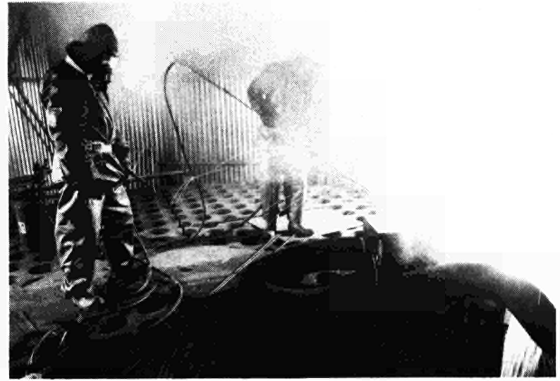
Figure 2: Cutting the Top Bioshield
