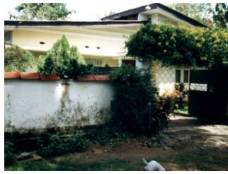
Houses with visual barrier
