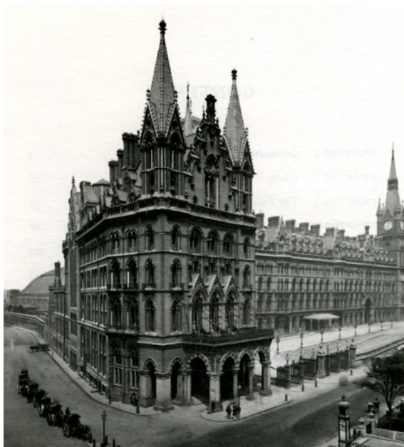
Figure 1. The Midland Grand Hotel at St Pancras Station, Euston Road, London, post 1874. © National Archive for Historic Decoration, University of Lincoln.
