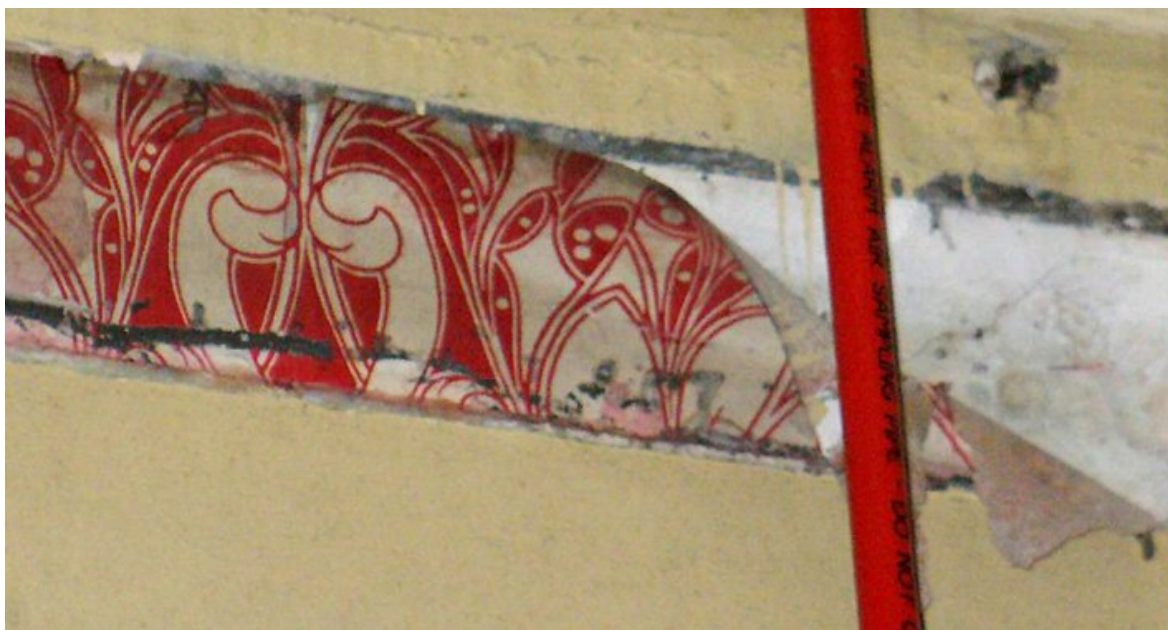
Figure 3 (above). Paper in the 3 rd floor corridor, exposed by removal of ducting, is very poorly attached to the wall. Figure 4 (left). Wallpaper from room 2.023 showing vertical staining pattern.
