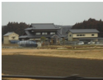
Evacuated buildings and tsunami damage observed from the vehicular survey
