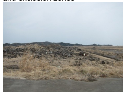
Tsunami damage observed from the vehicular survey
