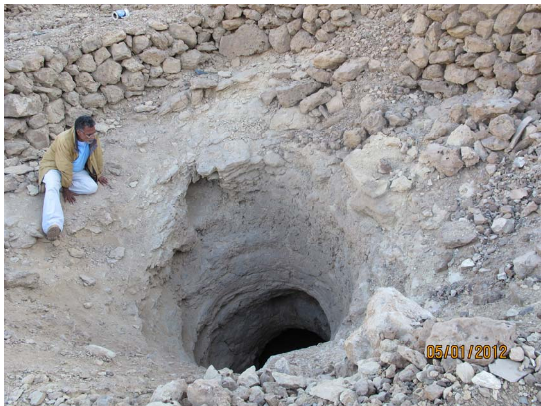
Fig. 56 - One of the shaft of the lead mine, protected by a stone wall (photo Pirelli)
