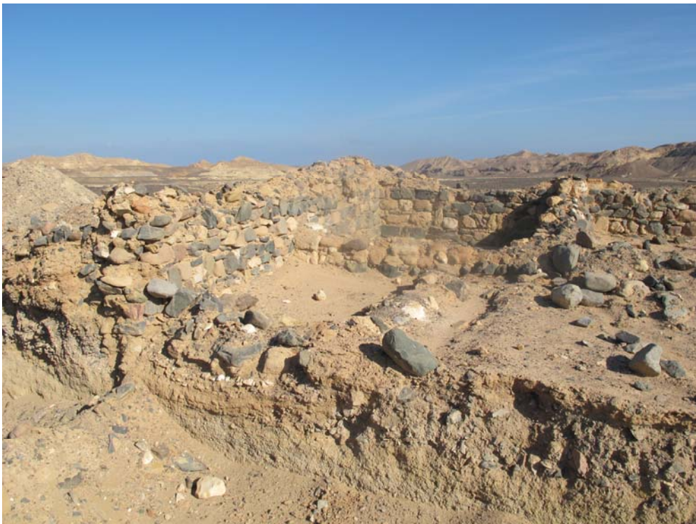
Fig. 35 - “Graeco-Roman Station”, Eastern building: foundation layers exposed by illegal excavation (photo Pirelli)
