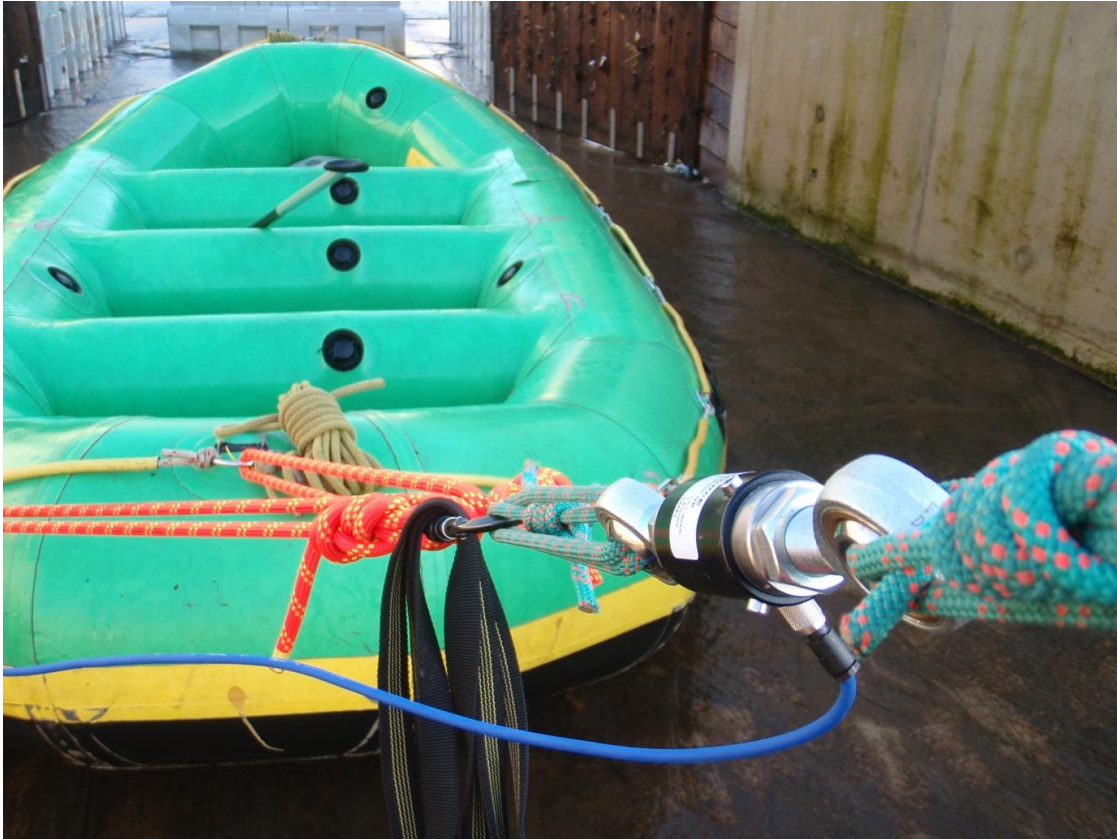
Figure 3. Force Logic Universal Load Cell and data cable positioned in between anchor leg focal point and connection to high line.
