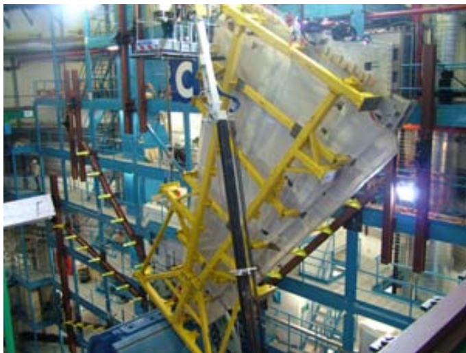
Figure 3.13: Installation of a part of one of the muon spectrometer wheels.
