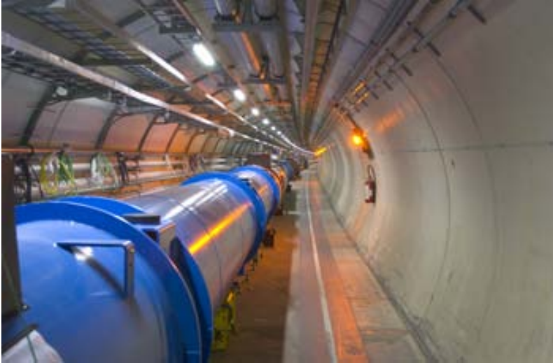
Figure 3.2: First dipole installed in the LHC tunnel in 2005.
