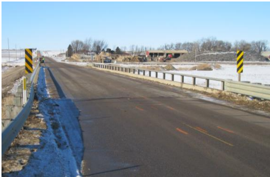
Figure 3. Sioux County Bridge end view
