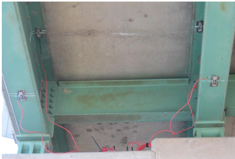
Figure 10. Sioux County Bridge instrumentation setup
