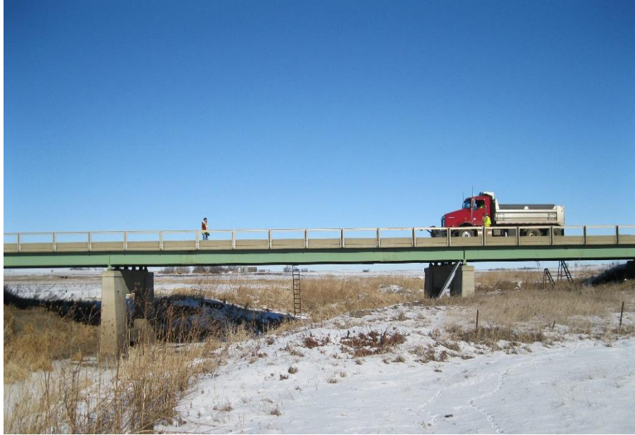
Figure 4. Sioux County Bridge elevation view
