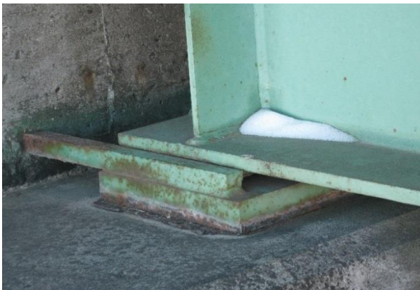
a. Abutment bearing
