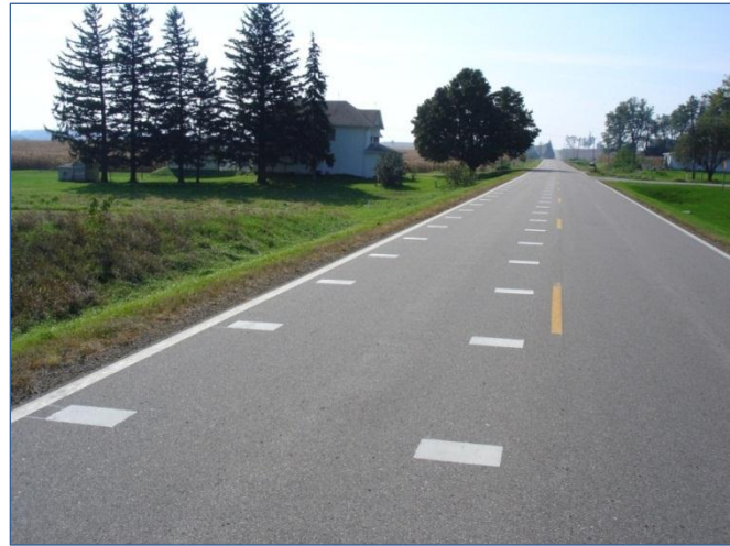
Figure 12. Transverse pavement markings as a rural gateway traffic calming treatment (Hallmark et al. 2007)
