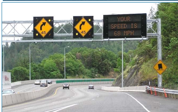
Southbound signs before and after
