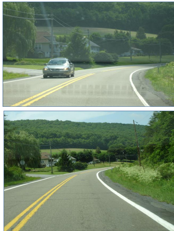
Figure 7. Before and after application of wider edge lines (Donnell et al. 2006)
