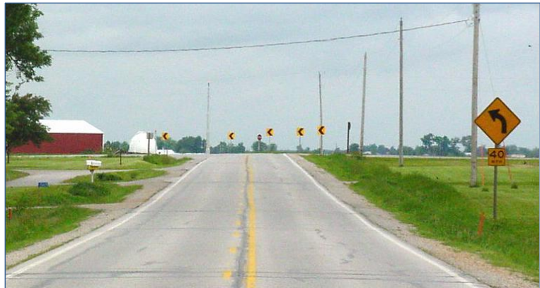
Figure 2. Oversized chevrons on US 6 in Johnson County, Iowa (Tom Welch, Iowa DOT)
