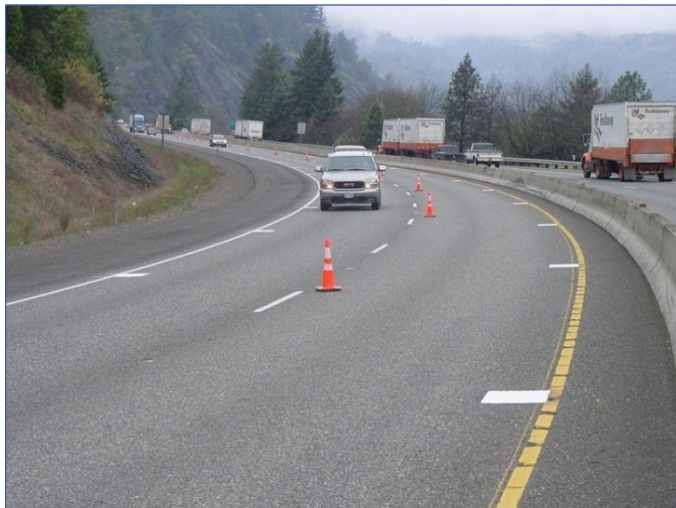
Figure 10. Optical speed bar installation on a curve in Oregon
