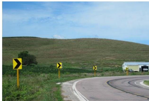
Figure 18. Delineator posts along a curve ( www.pexco.com/Pages/PexcoTrafficRDP.aspx )
