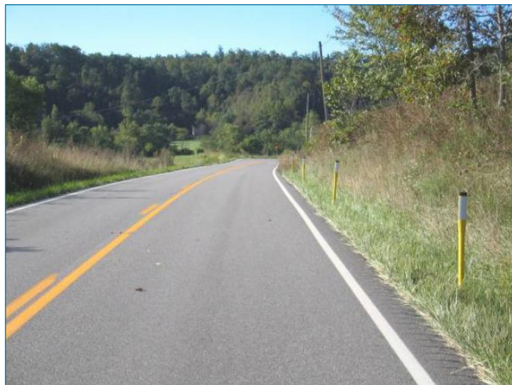
Figure 21. Post-mounted delineators at 50 ft intervals (Vest et al. 2005)
