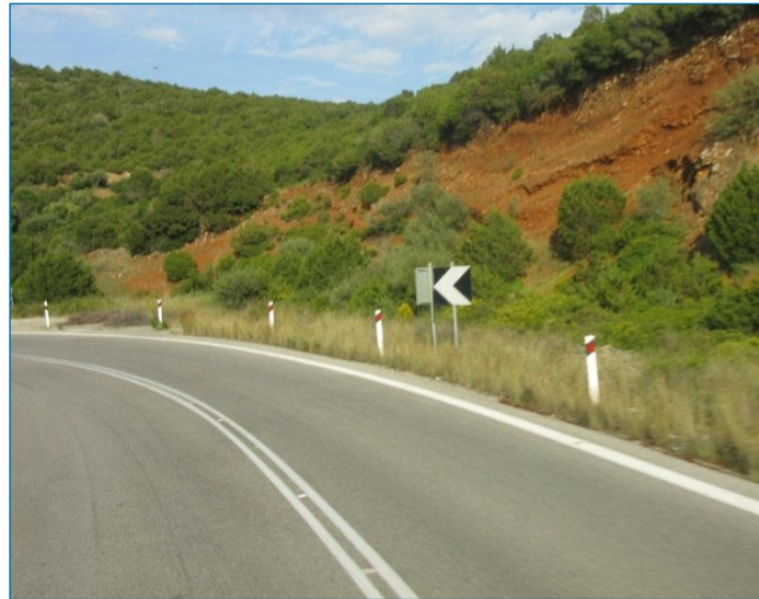
Figure 20. Post delineators on a curve
