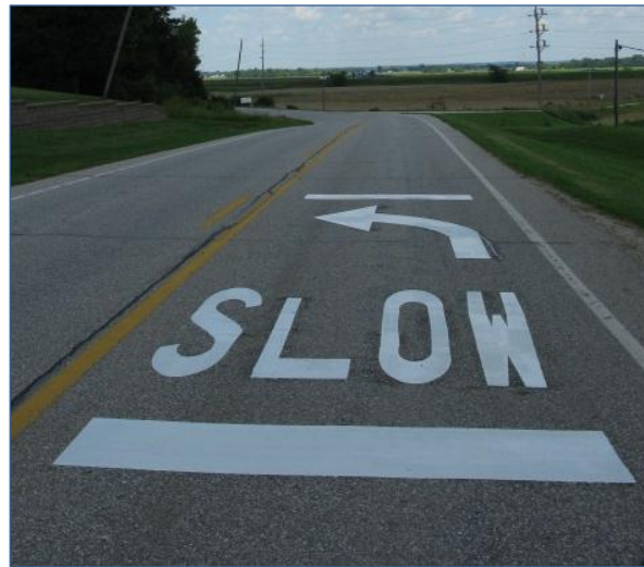
Figure 29. On-pavement curve sign
