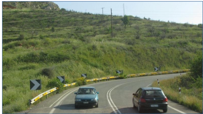
Figure 3. Panels of retroreflective sheeting to delineate curves
