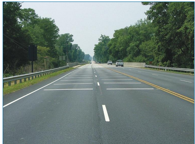
Figure 17. Transverse markings on US 460 (Arnold and Lantz 2007)
