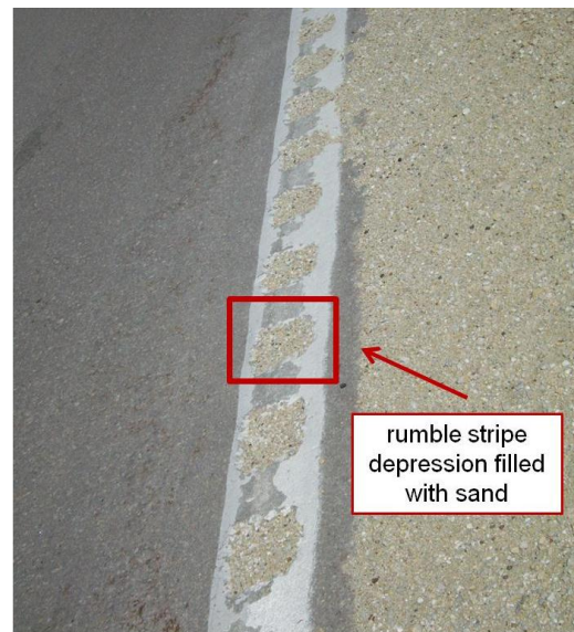
Figure 28. Rumble stripe depression filled with material (Hallmark et al. 2011)
