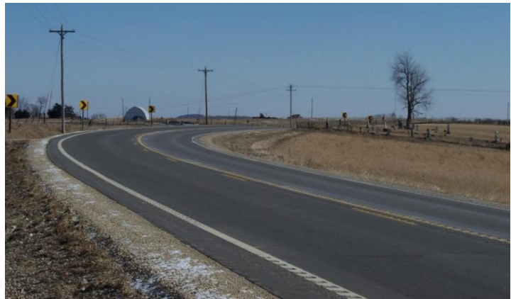
Figure 23. Edge-line and centerline rumble strips
