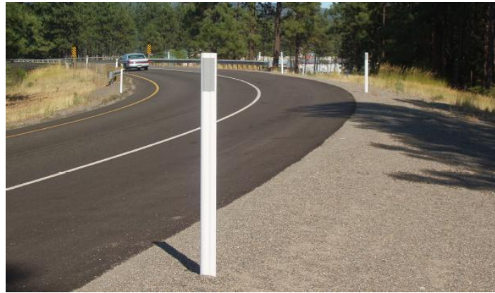
Figure 18. Delineator posts along a curve ( www.pexco.com/Pages/PexcoTrafficRDP.aspx )
