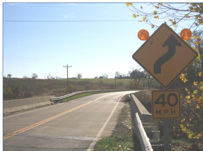
Figure 32. Flashing beacons on advisory curve sign (Vest et al. 20052)
