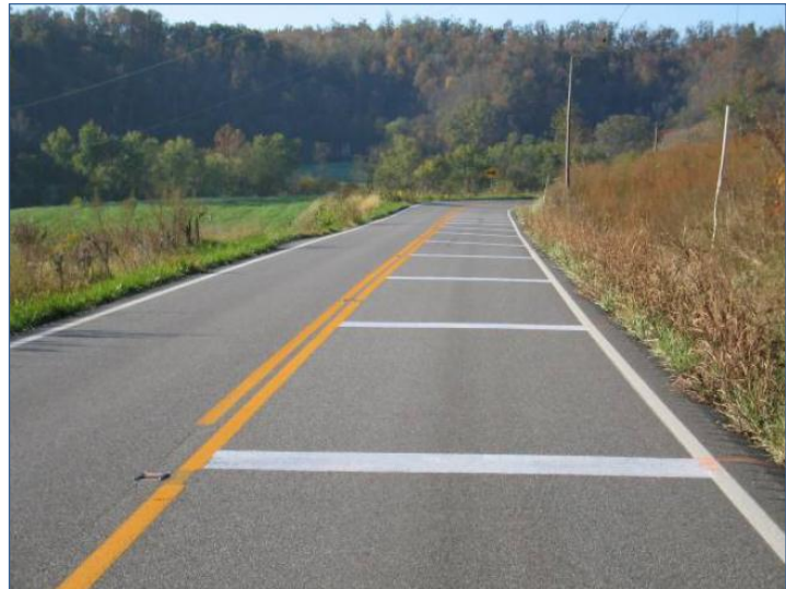
Figure 15. Equally-spaced transverse lines (Vest et al. 2005)
