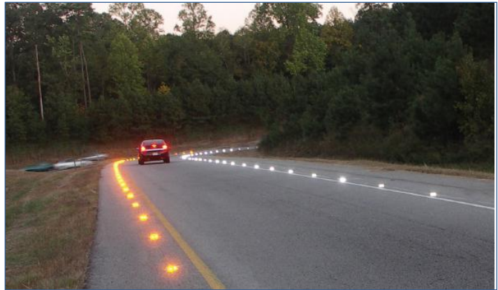
Figure 39. In-pavement lighting (FHWA 2011)
