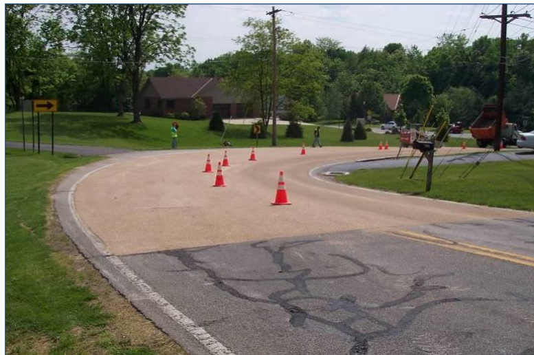
Figure 5. High friction treatment (The Transtec Group, Inc., highfrictionroads.com )
