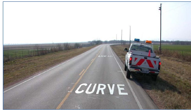
Figure 30. On-pavement curve markings (Chrysler et al. 2006)
