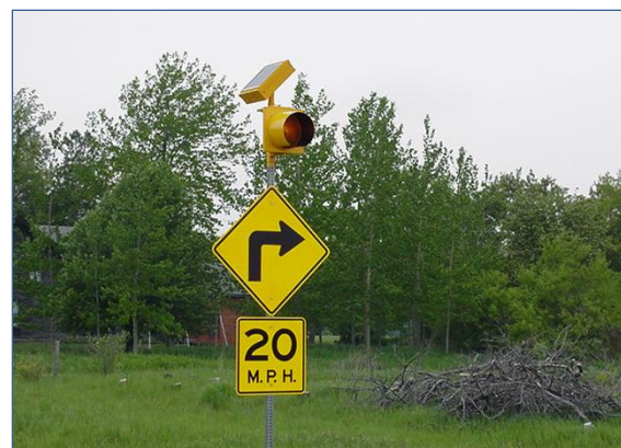
Figure 31. Flashing beacons (Bowman 2012)
