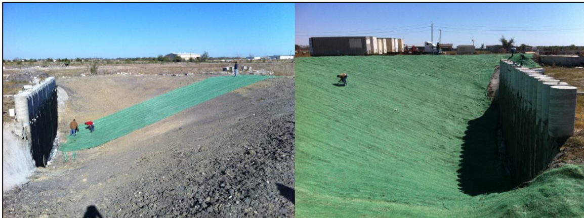
Figure 6.6: Erosion control material is installed on October 18, 2011.
