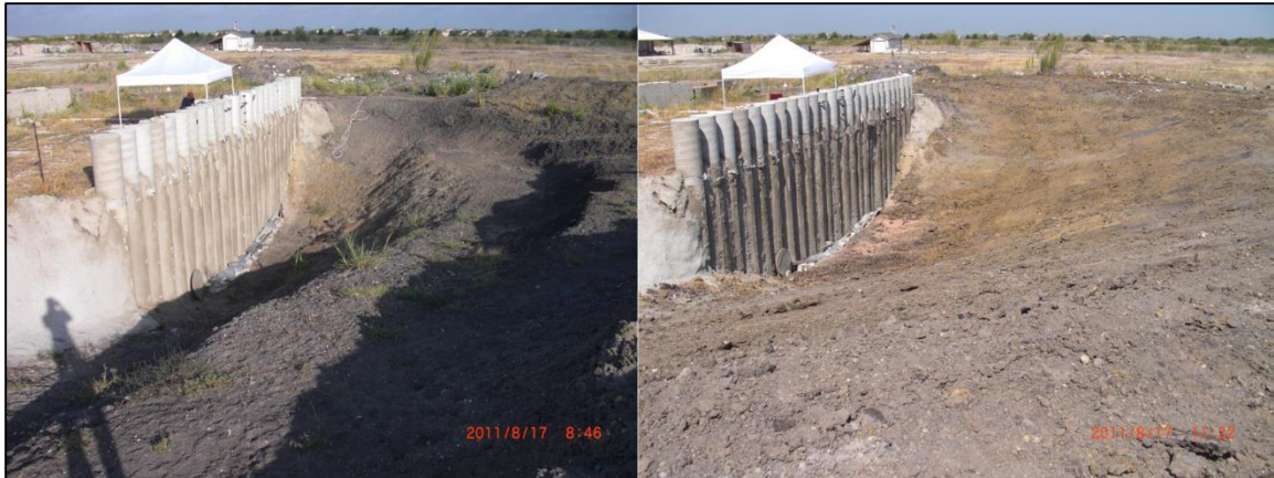
Figure 6.5: Excavation slopes are reshaped on August 17, 2011.
