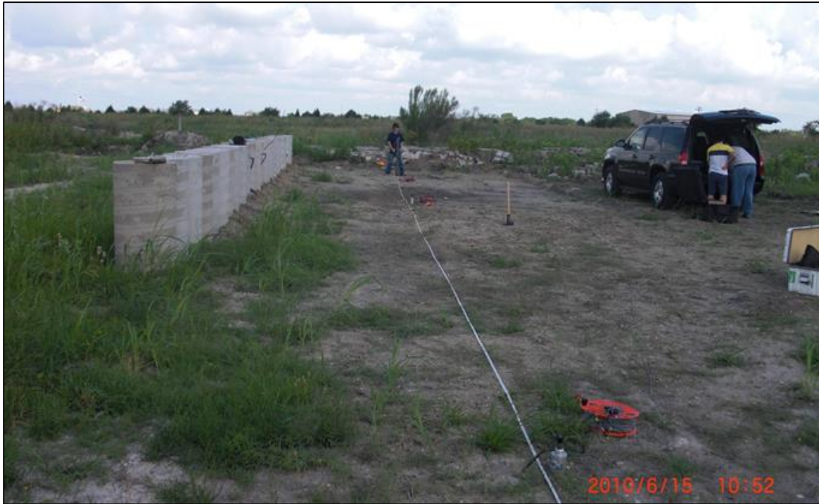
Figure 5.35: SASW testing at the test wall prior to excavation, June 2010.
