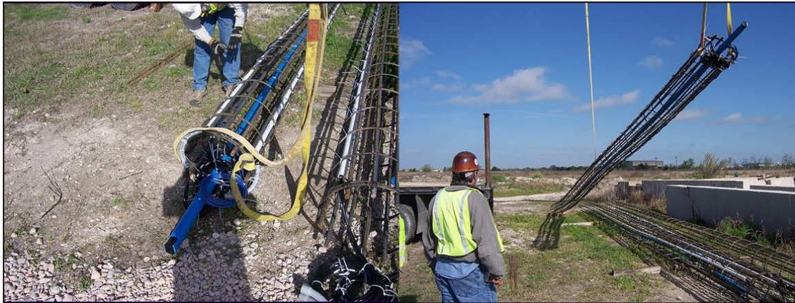
Figure 3.11: Lifting an instrumented cage with two cranes.
