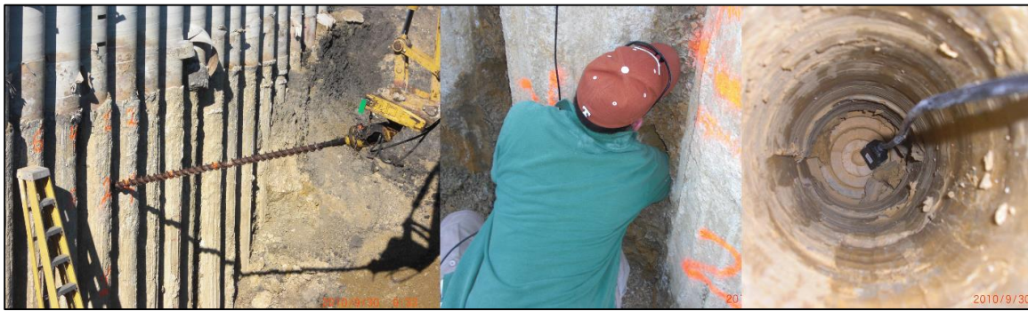
Figure 6.2: Installation of TDR Moisture Probes Behind Wall Facing.
