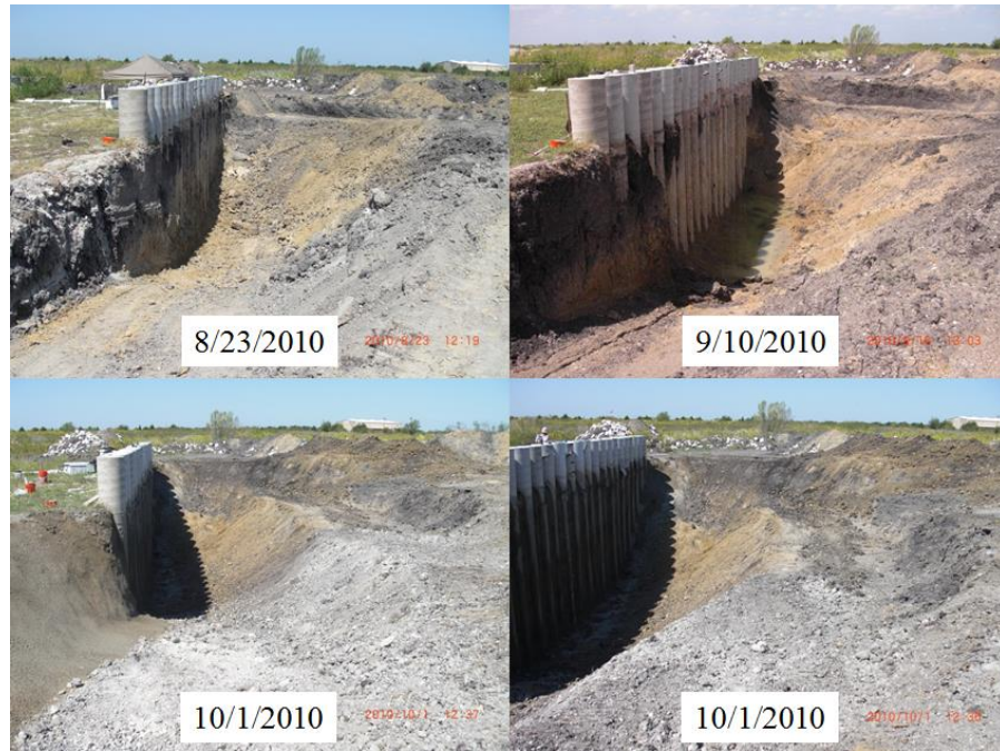
Figure 5.2: Photos of later excavation progress (8/23/2010 - 10/1/2010).
