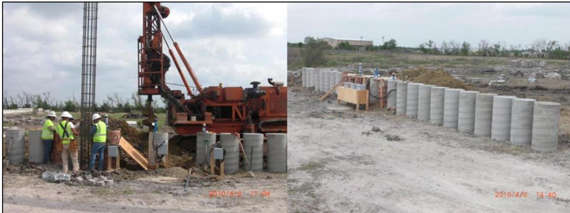
Figure 3.10: Construction of test wall, April 2010.
