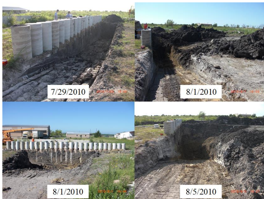
Figure 5.1: Photos of initial excavation progress (7/29/2010 – 8/5/2010).
