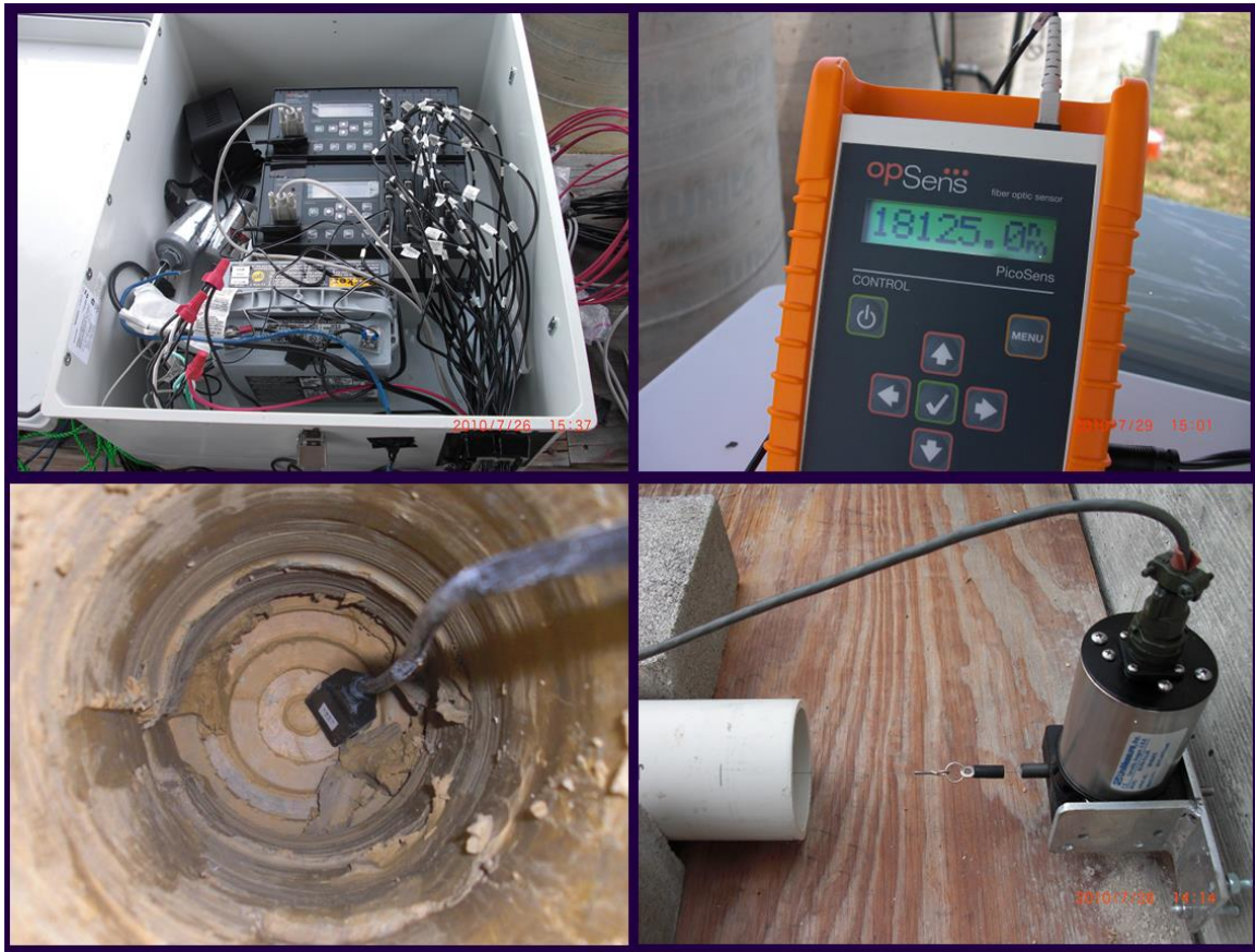
Figure 3.9: Instrumentation on the project site. Clockwise from top left: temperature resistant datalogger and enclosure for continuous strain readings; signal conditioner for individual strain readings; linear potentiometer; TDR probe installed through facing.
