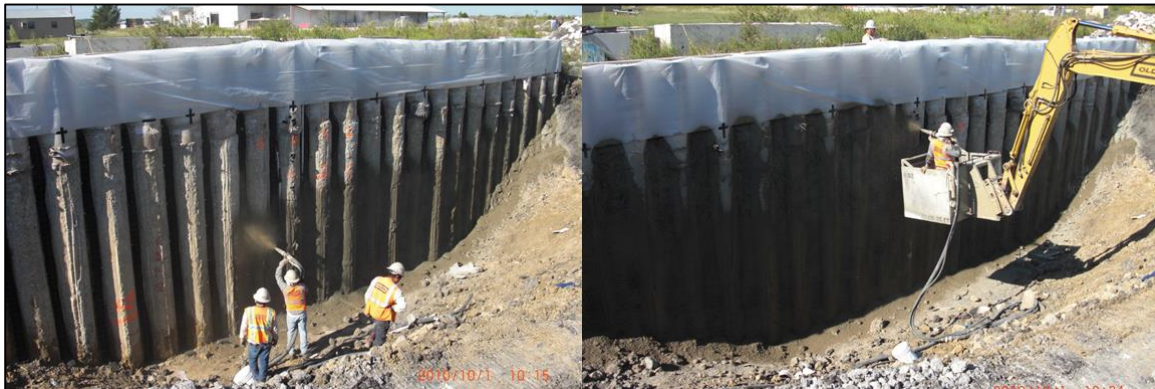
Figure 6.1: Installation of Shotcrete Facing on October 1, 2010.
