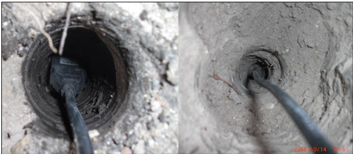
Figure 6.3: Installation of TDR Moisture Probes Through Ground Surface.
