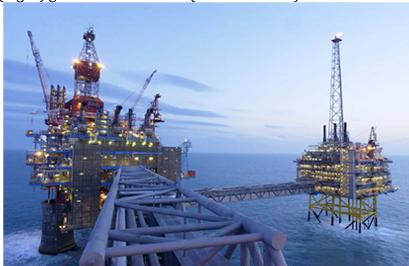
Fig. 9. A platform for injecting \text{CO}_2 into safe, geological storage: Sleipner, Norway. Courtesy of Statoil.
