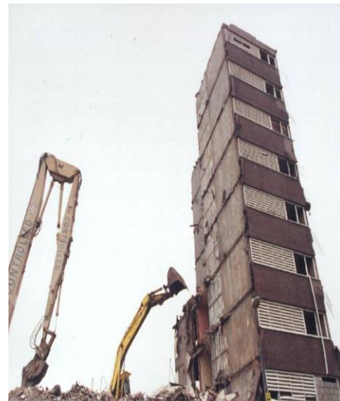
Figure 5.22: Demolition of the Centre 8 tower blocks
