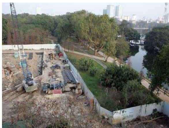
The hotel site under construction, February 2009 (LeN et al 2009)
