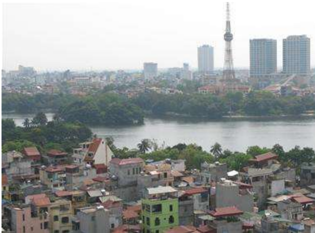
Reunification Park viewed from the southwest, with the Vincom Towers at upper right (source: http://tintuonline.com.vn )
