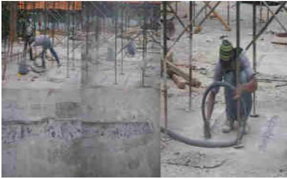
Figure 18. Implementation process and results Patching
