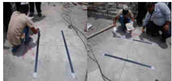
Figure 20. CFRP installation process
