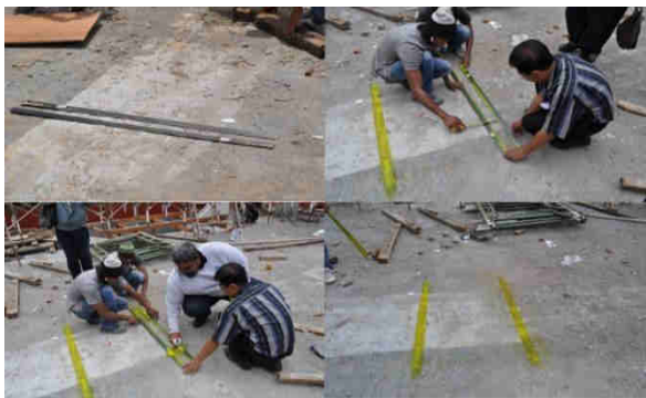
Figure 19. Implementation of Measurement and concrete surface markings
