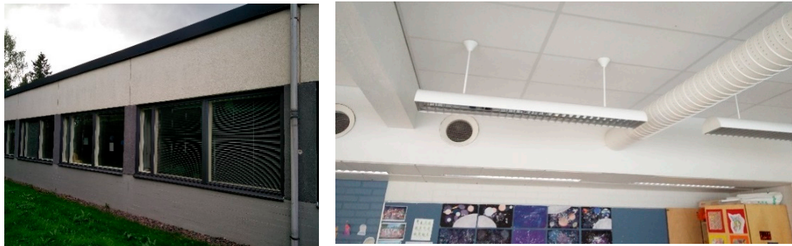
Figure 1. Studied building section, a typical supply air duct diffuser, and an extract air grille in a classroom.
