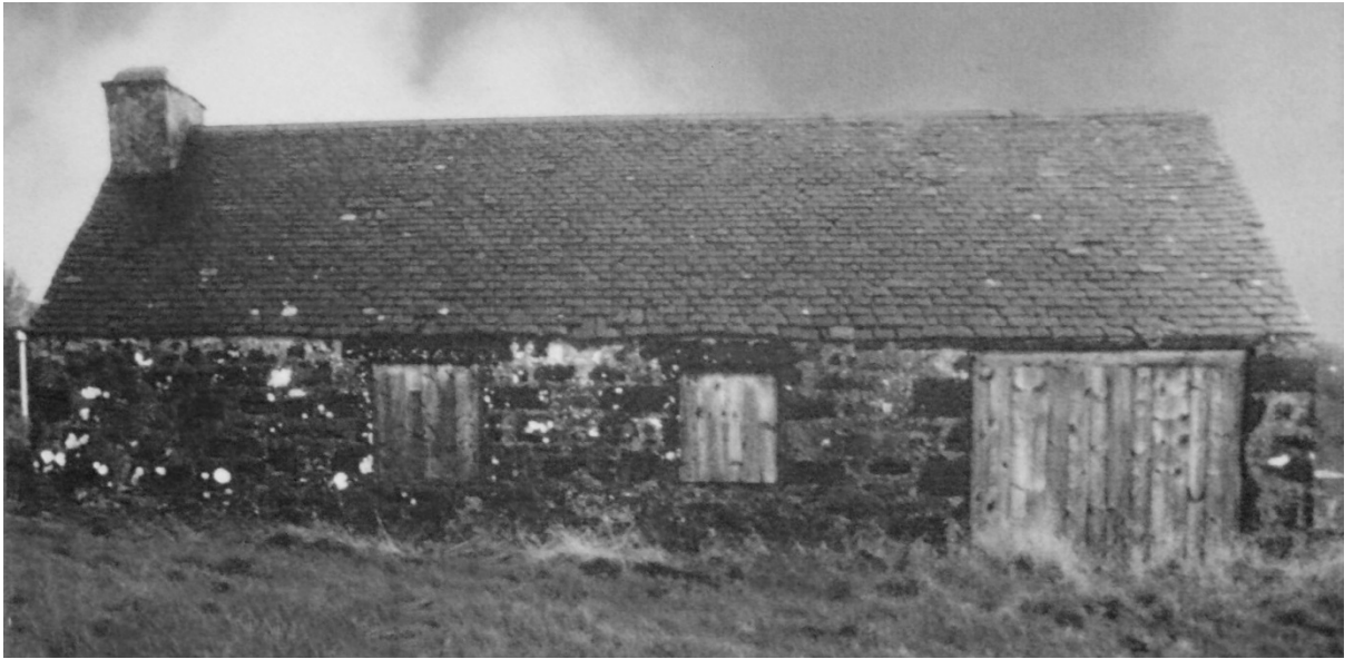
Figure 1. View of former Smithy, now LSIC building, from the west.
