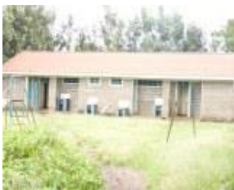
Photo 7.1 Toilet block (L) at Boonhouse
