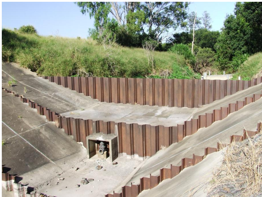
Figure 90. Laidley diversion weir in 04/2008. Dry creek, no-flow period.
