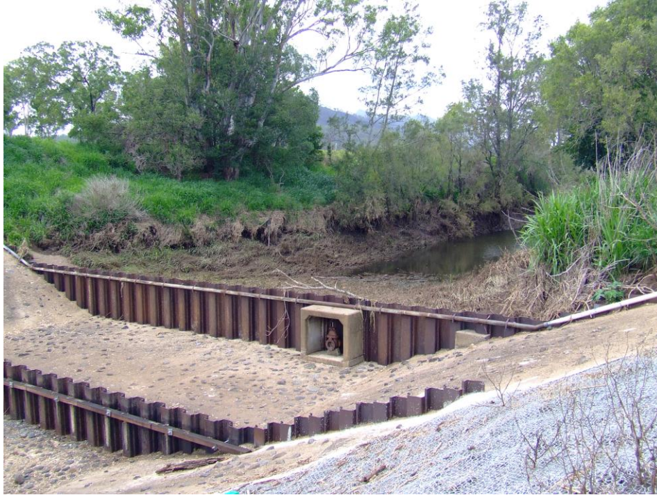
Figure 93. Mulgowie recharging weir in 11/2007. 24 hours after minor flood event, the water disappeared from the creek into the alluvial aquifer.
