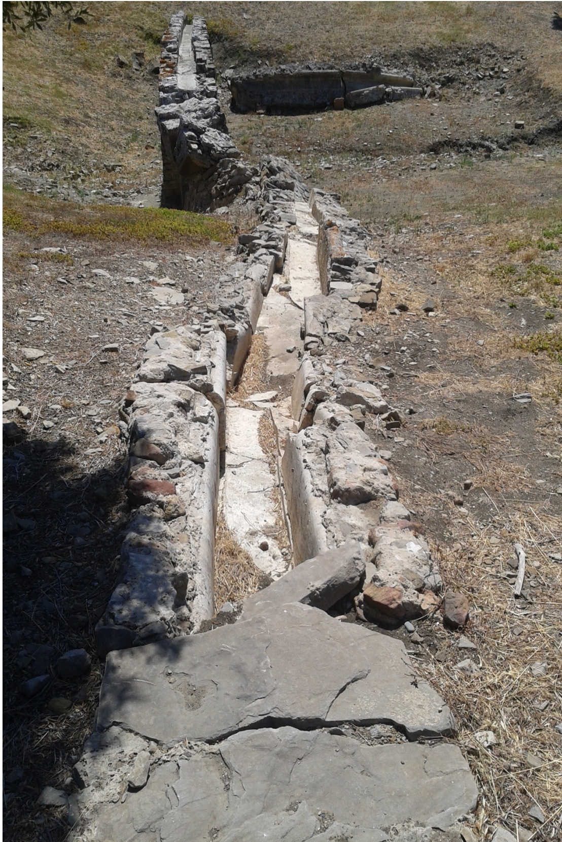
Figure 3: Broken remains of one of the aqueducts of Baelo Claudia (Cádiz), damaged by an earthquake in the third century and never repaired (photo by Elena Sánchez).
