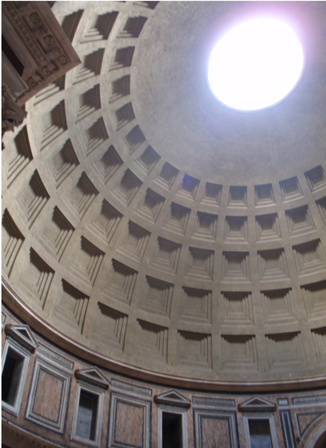
Figure 1: The Pantheon in Rome, with its concrete dome and brick rotunda, is one of the feats of Roman engineering (photo by the author).
