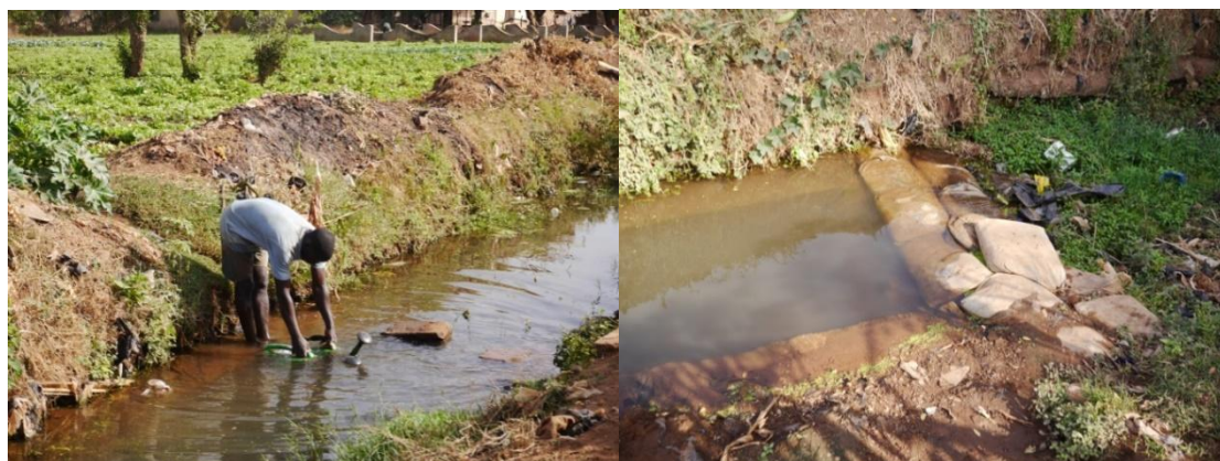
Figure 6.10: Water source at Gumbihini waterworks
