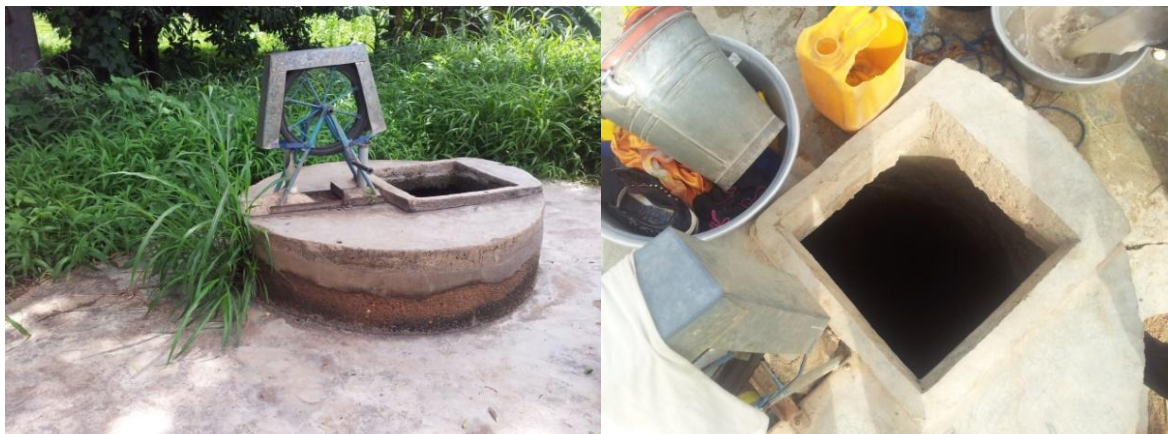
Figure 6.11: Well installed by New Energy in Zagyuri vegetable site
