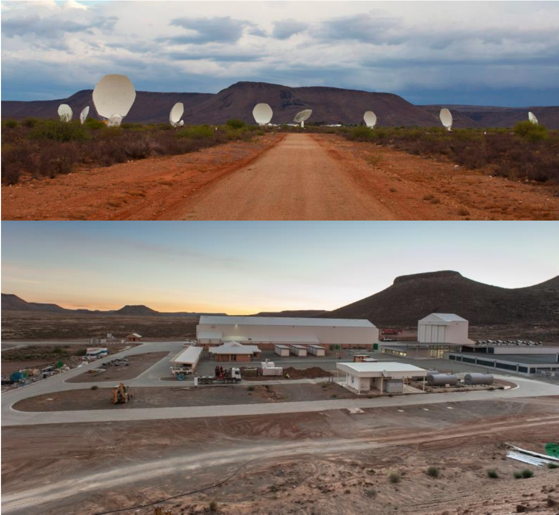
Figure 3.1: development of the MeerKAT telescope array and KAPB construction[86]
